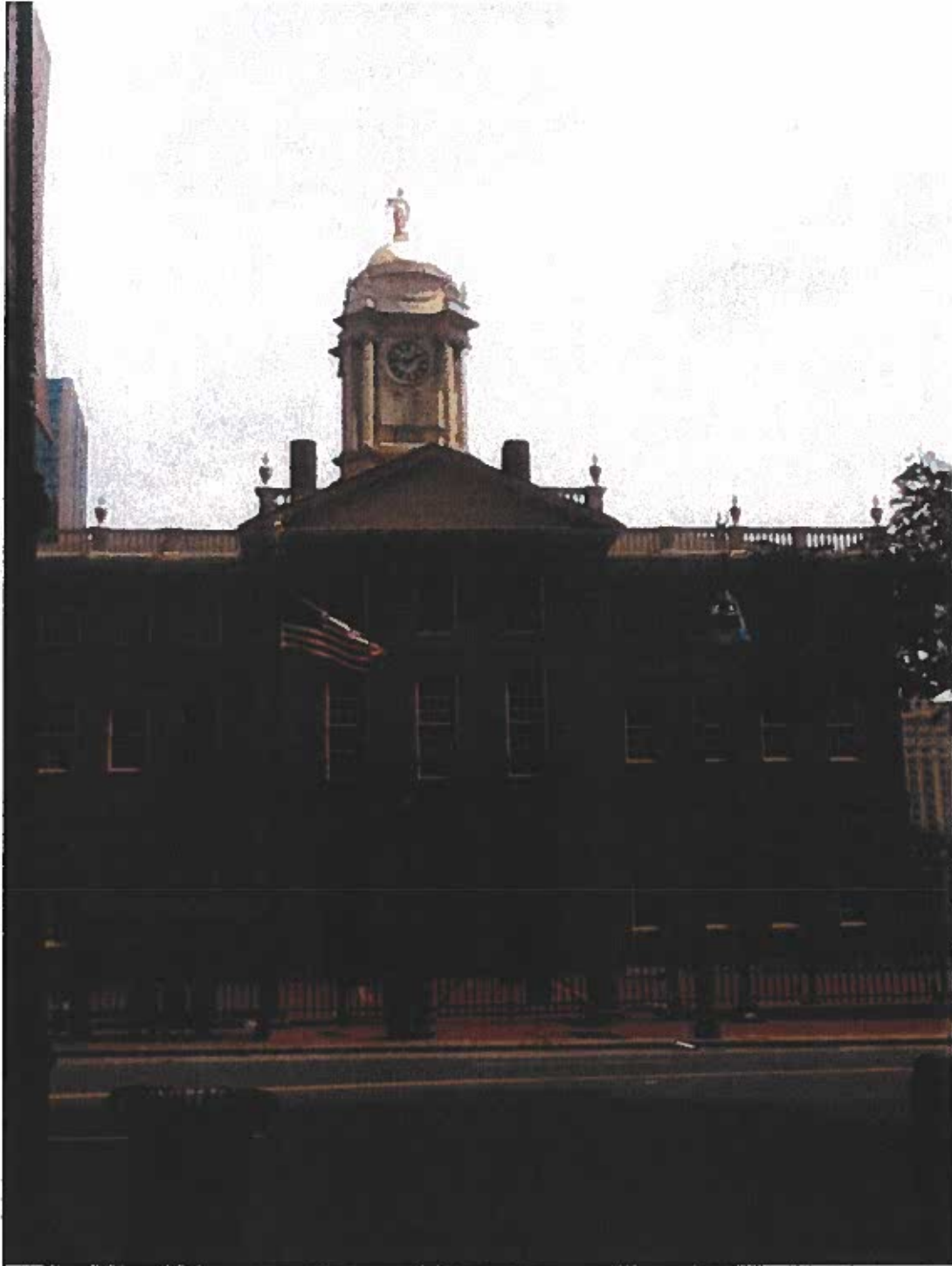
HISTORICAL REFERENCE - STATE HOUSE - BLACK METAL RAILING -
