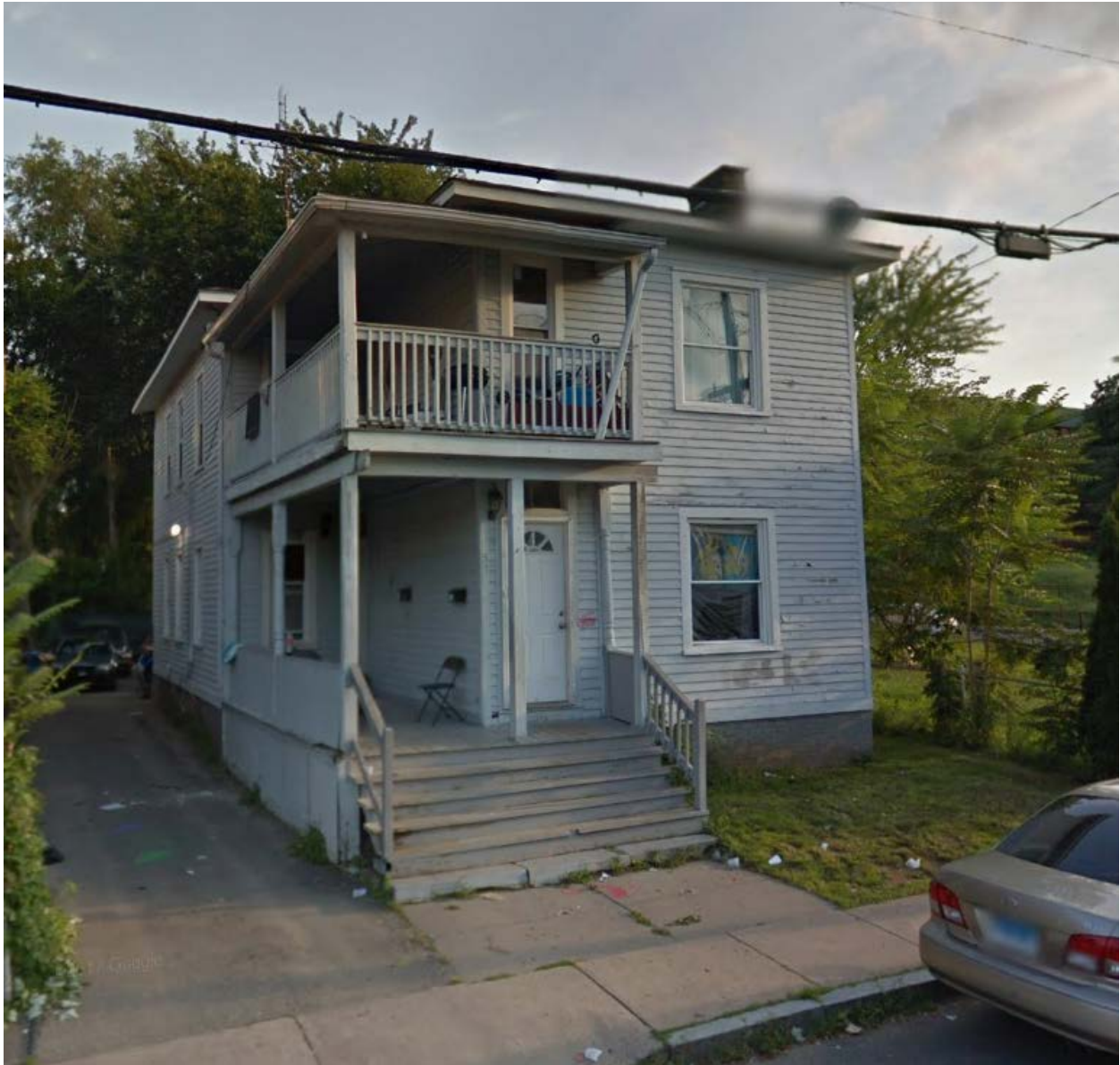
53 Grand Street, Google street view June 2017
