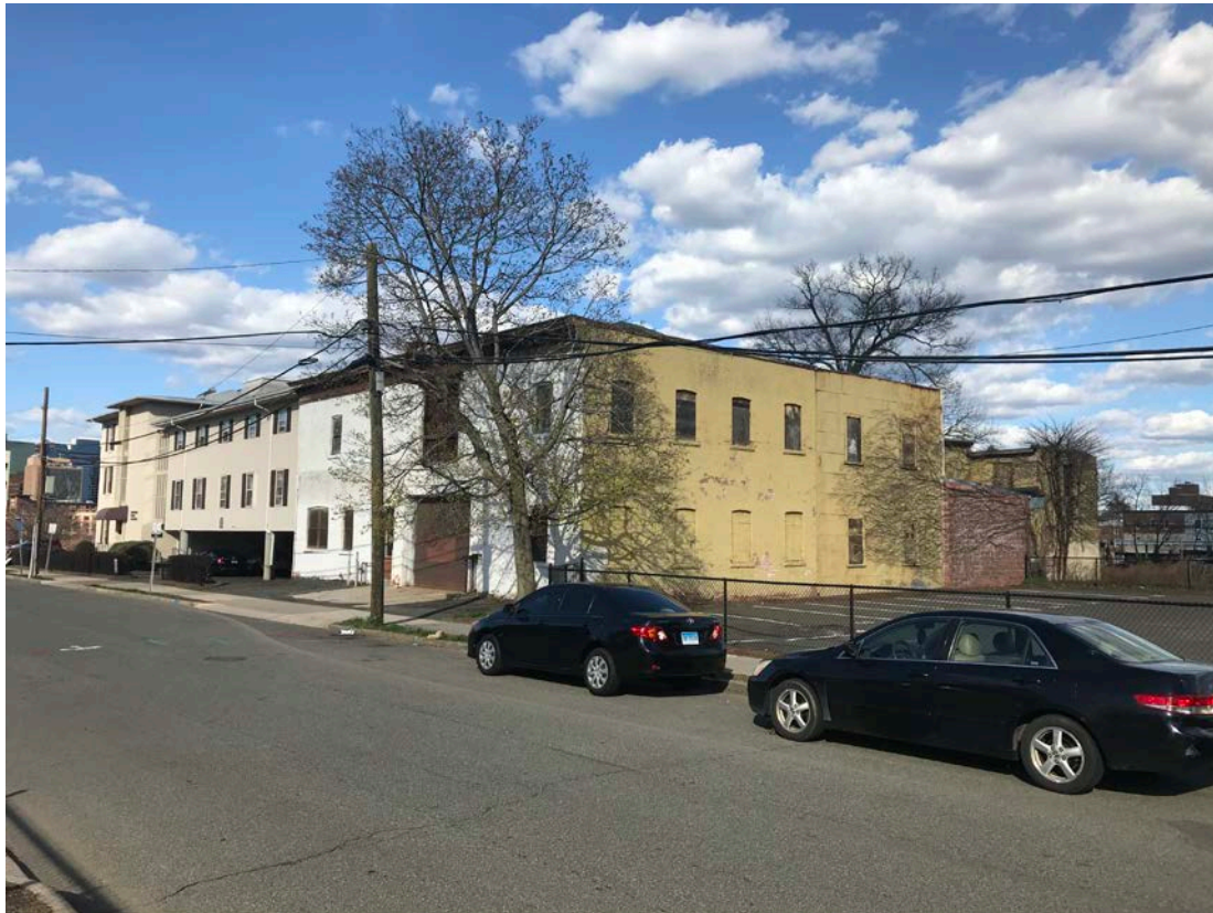
Fig.1 - 100 Cedar Street Front and Side (south) façade taken on April 13, 2021
