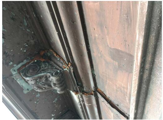
Corbel appears to have fallen off and been refastened. Gaps created by movement have been filled with expanding foam insulation. Soft wood behind the metal was observed in this area
