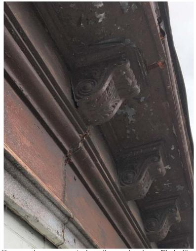
Another joint with excessive movement where the gap has been filled with expanding foam insulation. Note the gaps at the corbel and between the wall and the cornice.
