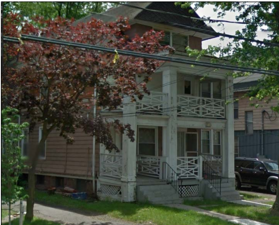
Picture-2, Old photo of front porch steps with metal guardrails
