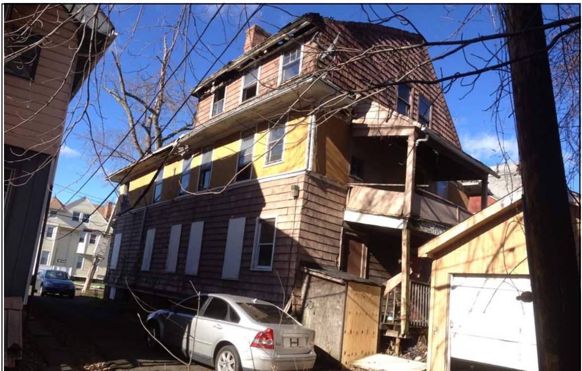
Picture-4 North side looking South/West
