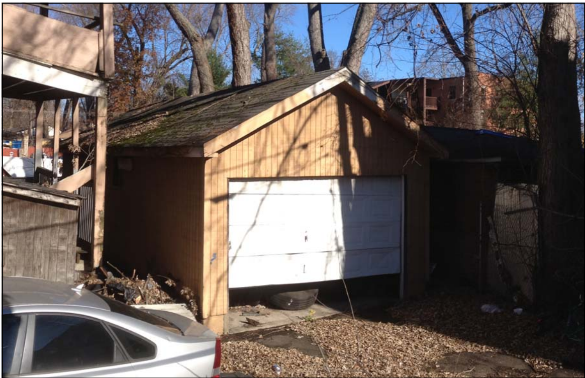
Picture- 6 Garage at rear of property
