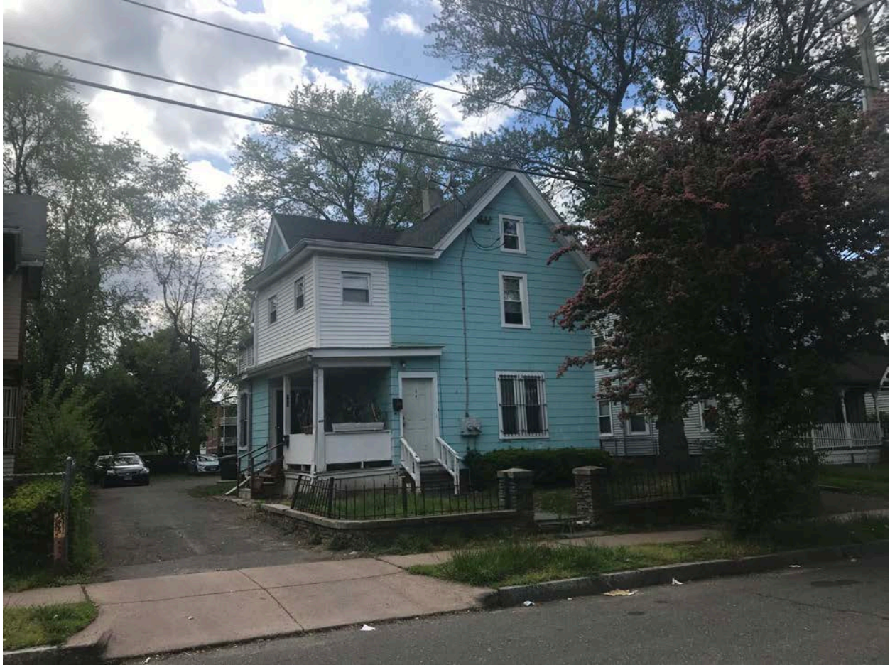
Side (South) and Clark Street (East) Facades – Photo taken 5/13/21
