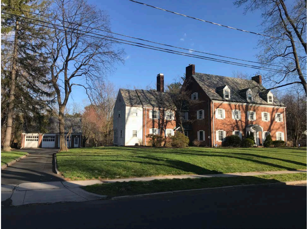
Fig. 1 - Front and Side (North) Façade of 222 Girard Avenue taken April 13, 2021
