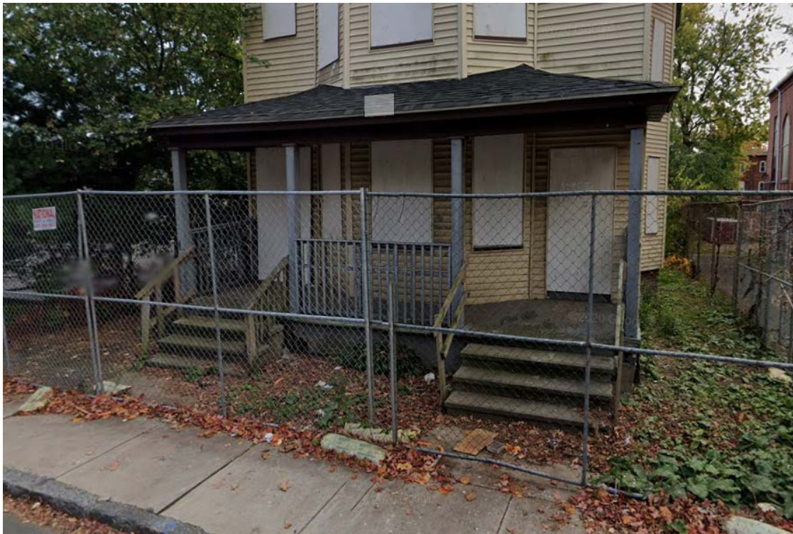
Fig. 2 - 29 Mather – Front Porch – Google Streetview, October 2020
