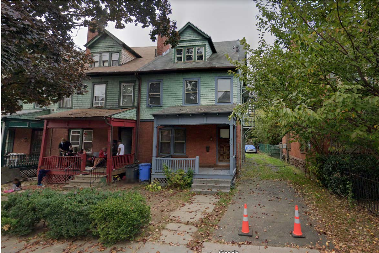
Fig. 1 - Front Façade – Google Streetview Image, October 2020
