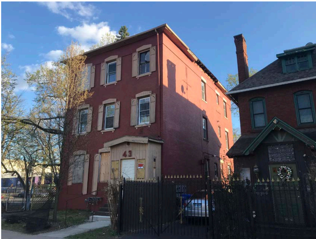
Fig. 1 - Front and Side (west) Façade - Photograph taken April 13, 2021
