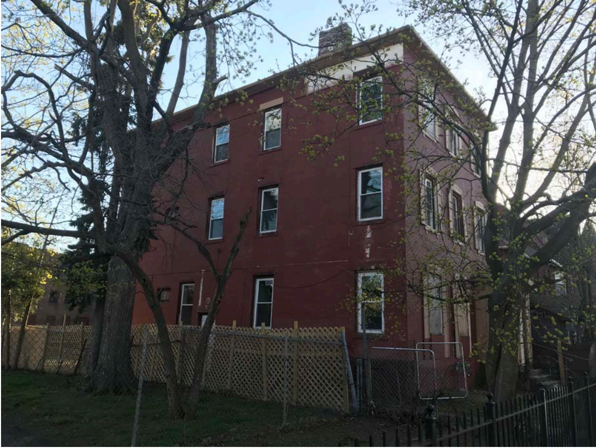
Fig. 2 - Side (east) Façade - Photograph taken April 13, 2021
