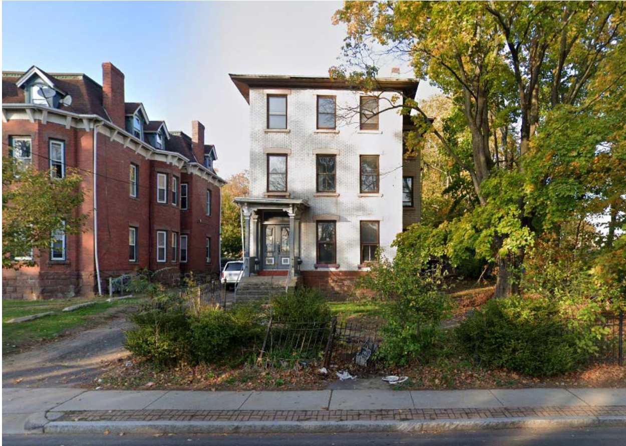
Fig. 1 - Front Façade – Google Streetview Image, October 2020
