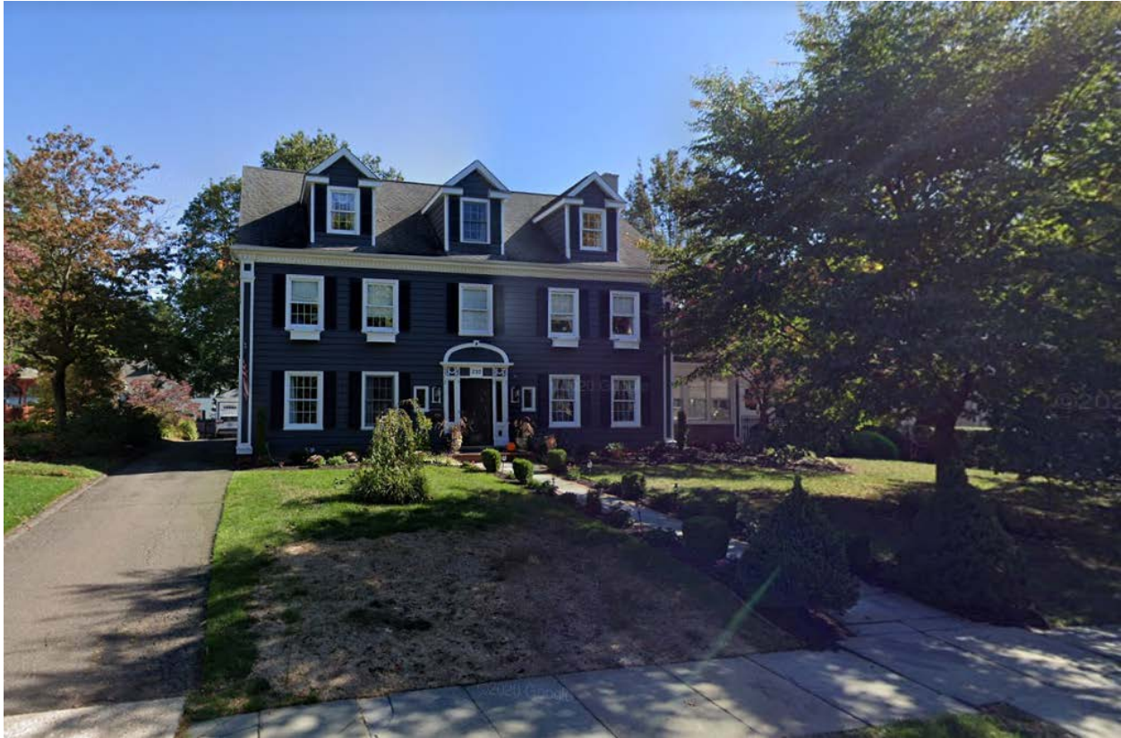
Front Façade from Kenyon Street – Google Street View Image October 2020
