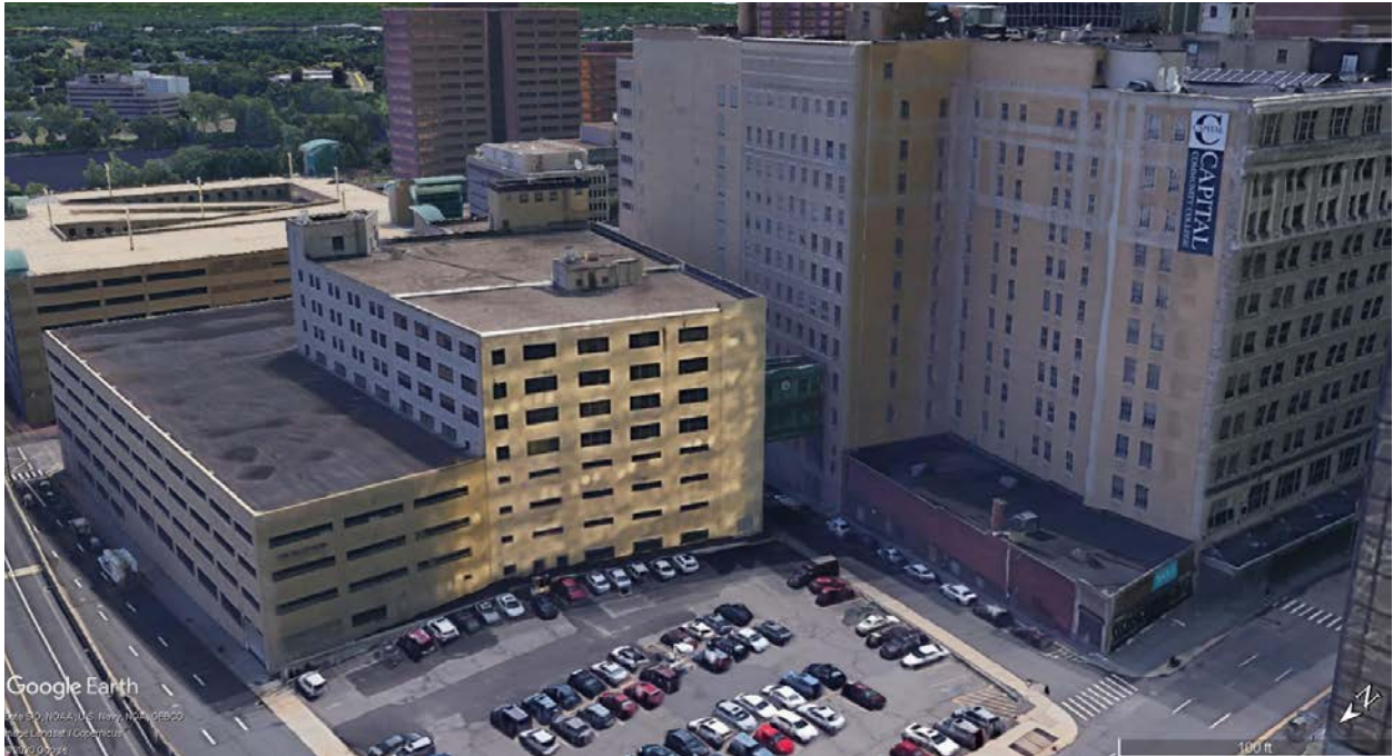
Figure 1. Google Earth, dated 9/18/2019. View of the 36-70 Talcott Street the intersection of Main and Morgan. The original warehouse structure is located along Talcott Street, in the center of the image, and the copper, Neoclassical Revival bridge connects it to the former G. Fox Store on the right, now Capital Community College. The 4-story addition on the left that wraps the north and east sides of the Warehouse Building is not within the district.
