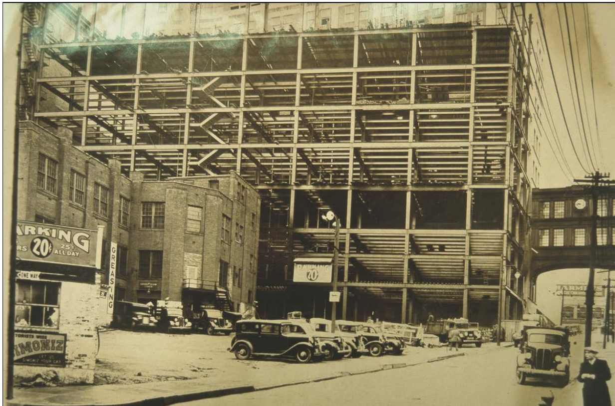
Figure 7. Unknown photographer, "G. Fox Store, Hartford: Exterior view, 1938 addition construction [HSP 2485]." doi:10.2307/community.159454. Trinity College's collection of Hartford images holds this photograph taken during construction of an eastern addition to the G. Fox. Store building and shows a portion of the pedestrian bridge.
