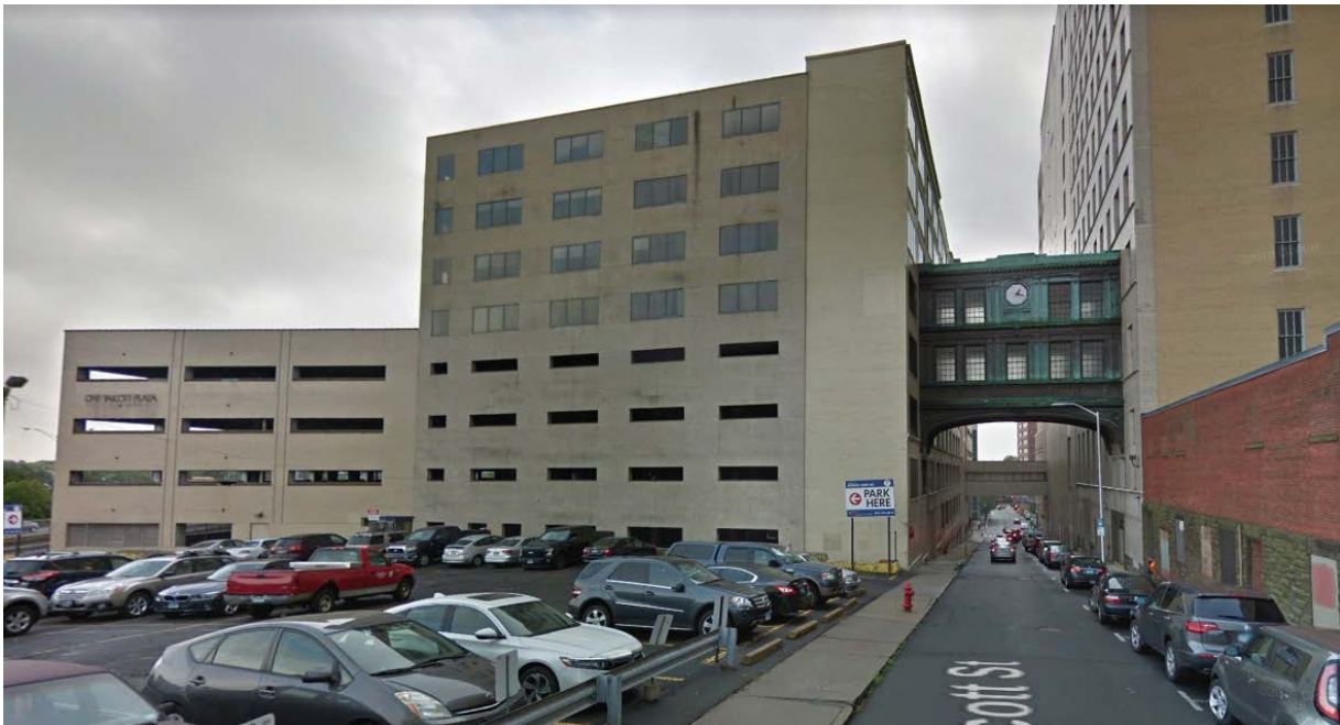
Figure 4. Google Streetview, dated June 2019. View east on Talcott Street from Main Street. The bridge is connected to the 1918, former G. Fox & Co. store building which is also of Neo-Classical Revival Style with Art-Deco marquisse added above first story (1935, Taussig-Flesch Associates) and further addition to the rear and upper stories.
