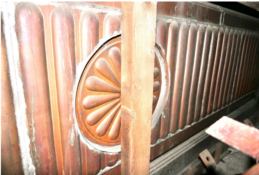
Figure 12. Original copper surfaces are visible behind interior wall access panels, on the first level, on the interior of the bridge where these surfaces were not exposed to weathering.
