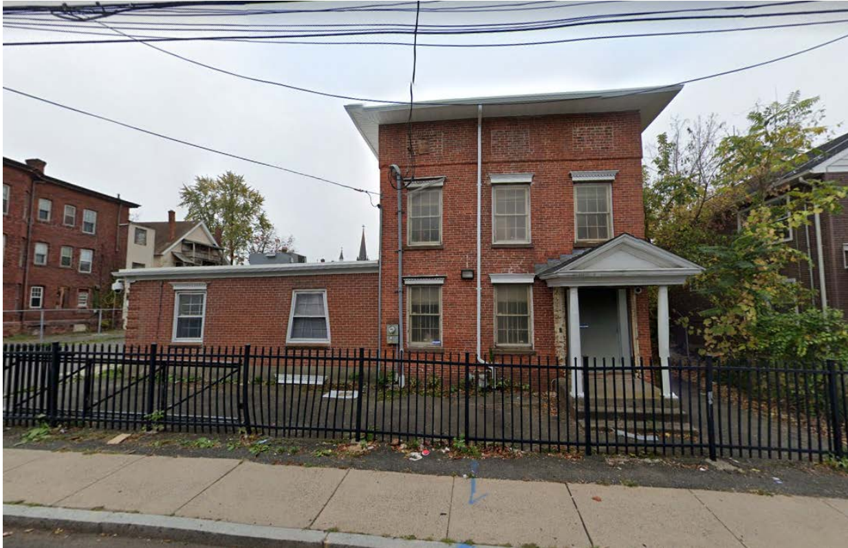
Fig.1 - Front Façade from Grand Street – Google Street View Image October 2020
