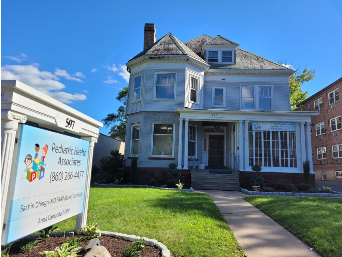
Figure 2. 597 Farmington Avenue – Staff Photo – August 6, 2021
