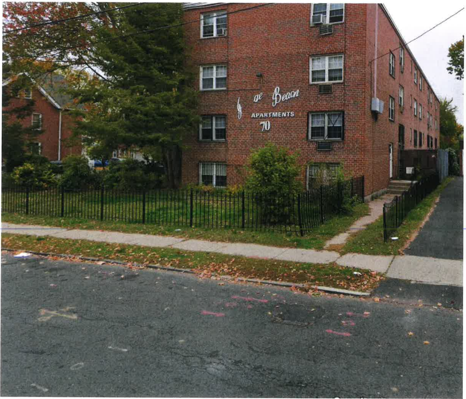
70 Allen Place, existing condition.
