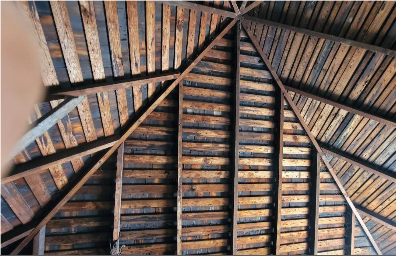
PHOTO #1 INTERIOR VIEW OF PYRAMID HIP ROOF.
