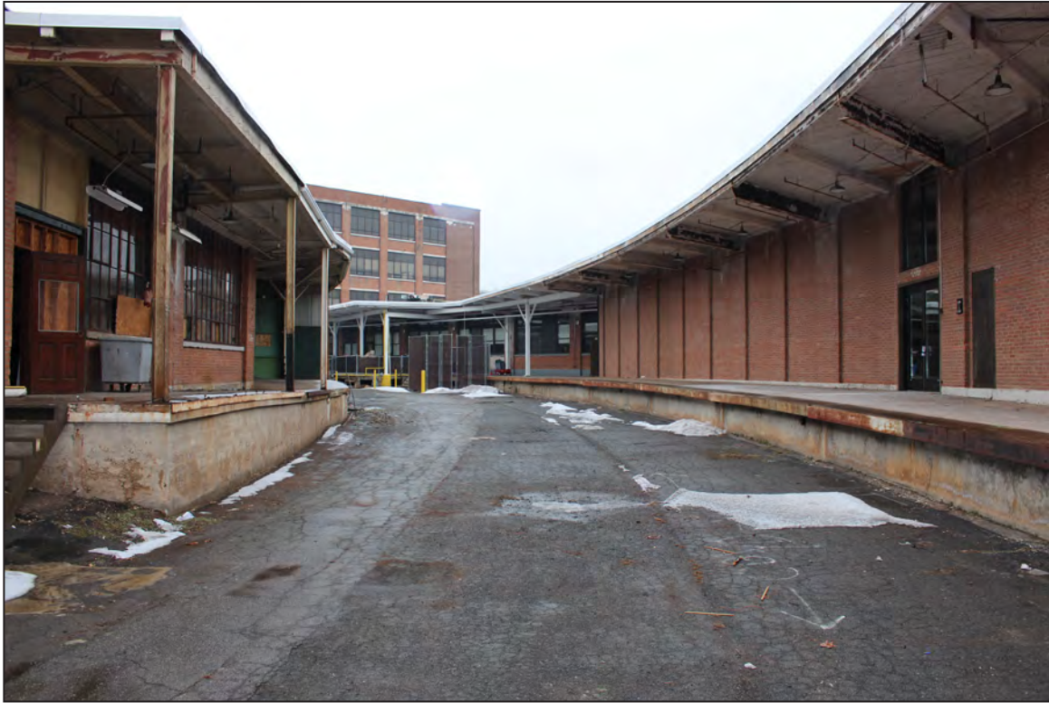
43. Site View, looking northwest. Factory/Warehouse Building (right) and Factory/Garage Building (left).
