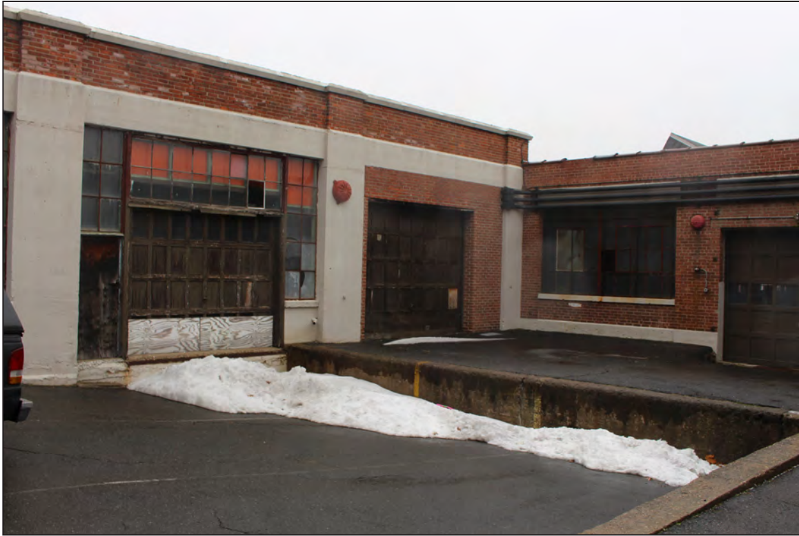
57. Factory/Garage Building, South and West Elevations, looking northeast.
