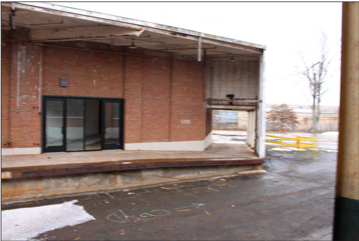
42. Factory/Warehouse Building, South Elevation, looking north.
