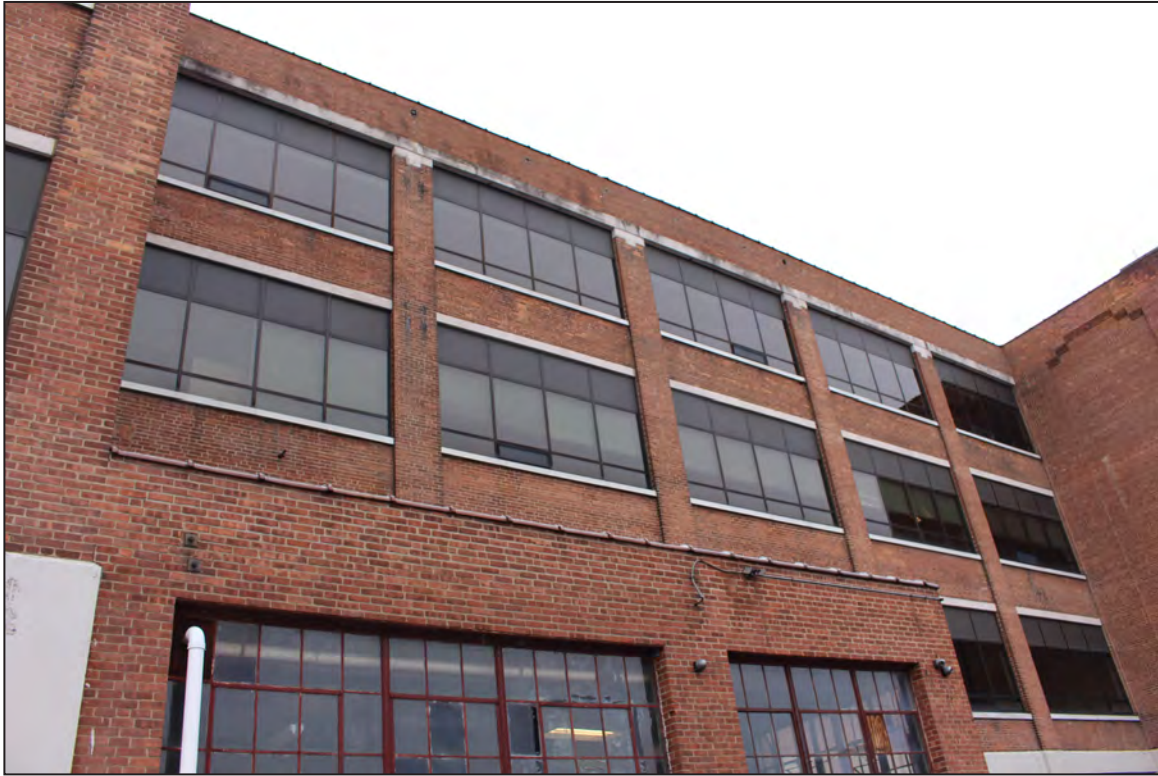
67. Main Office/Factory Building, East Elevation, looking northwest.
