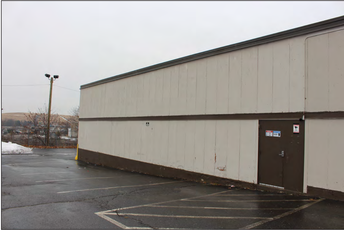
35. Factory/Warehouse Building, North Elevation, looking southeast.
