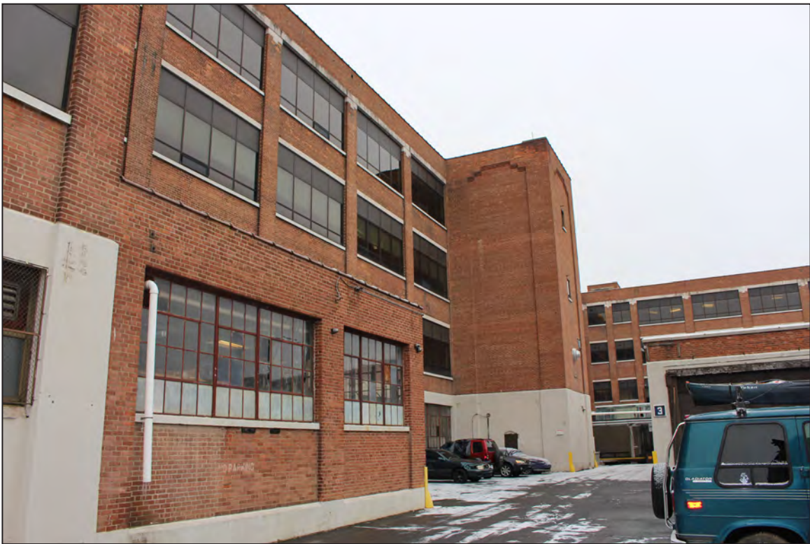
66. Main Office/Factory Building, East Elevation, looking northwest.
