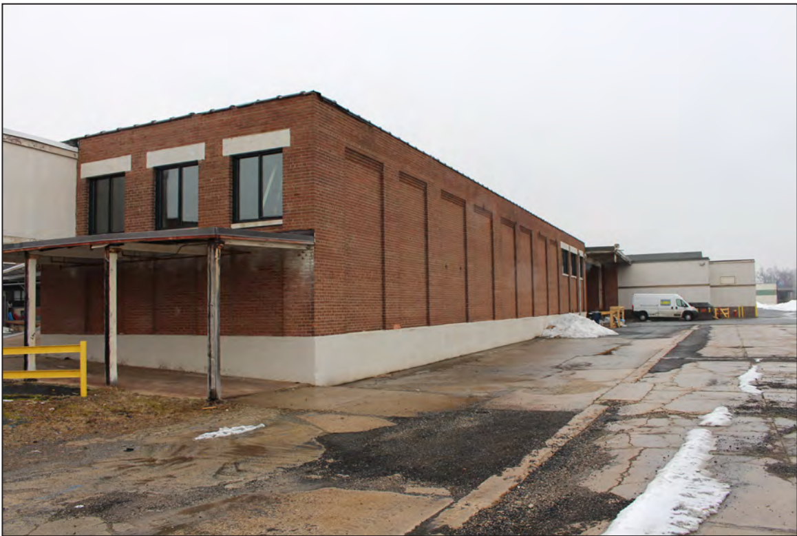
36. Factory/Warehouse Building, East Elevation, looking northwest.
