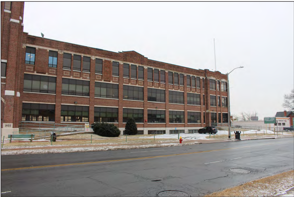
8. Main Office/Factory Building, West Elevation, looking southeast.
