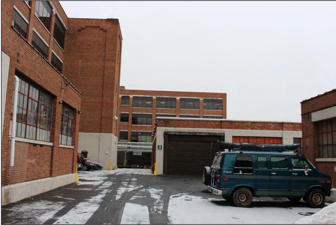
65. Site View, looking north. Main Office/Factory Building (left), Factory/Garage Building (right).
