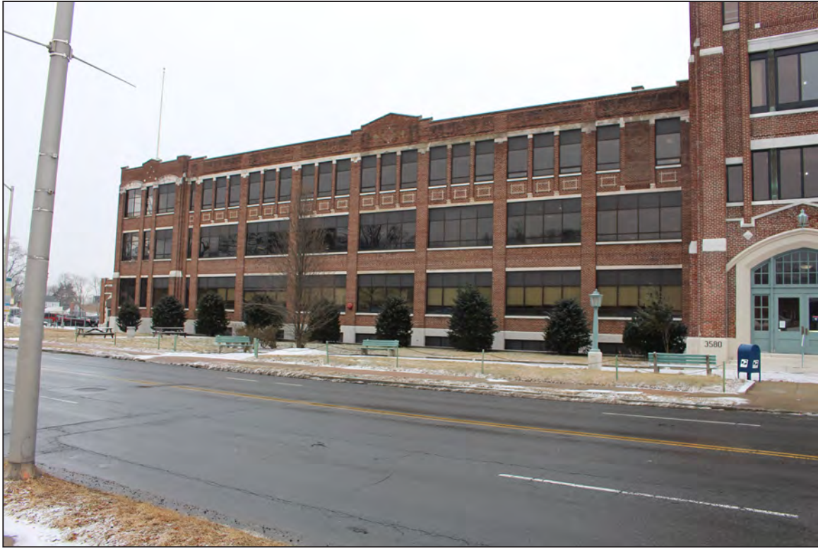
7. Main Office/Factory Building, West Elevation, looking northeast.
