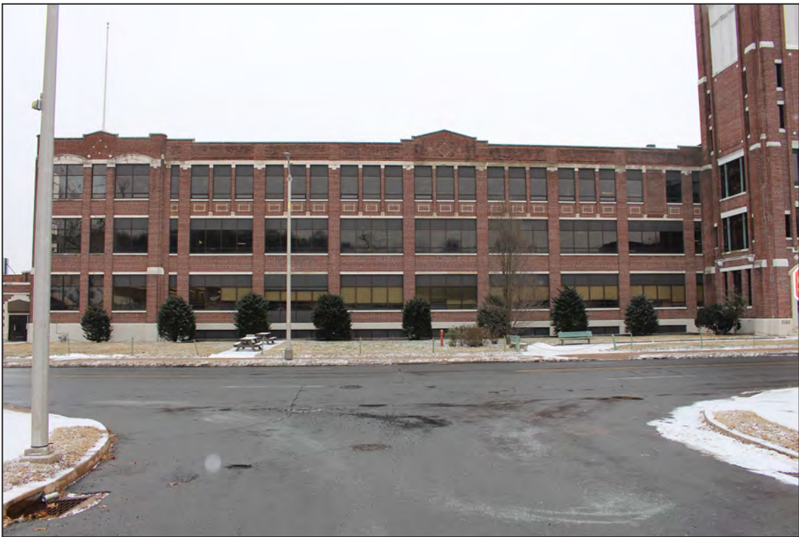
18. Main Office/Factory Building, West Elevation, looking east.
