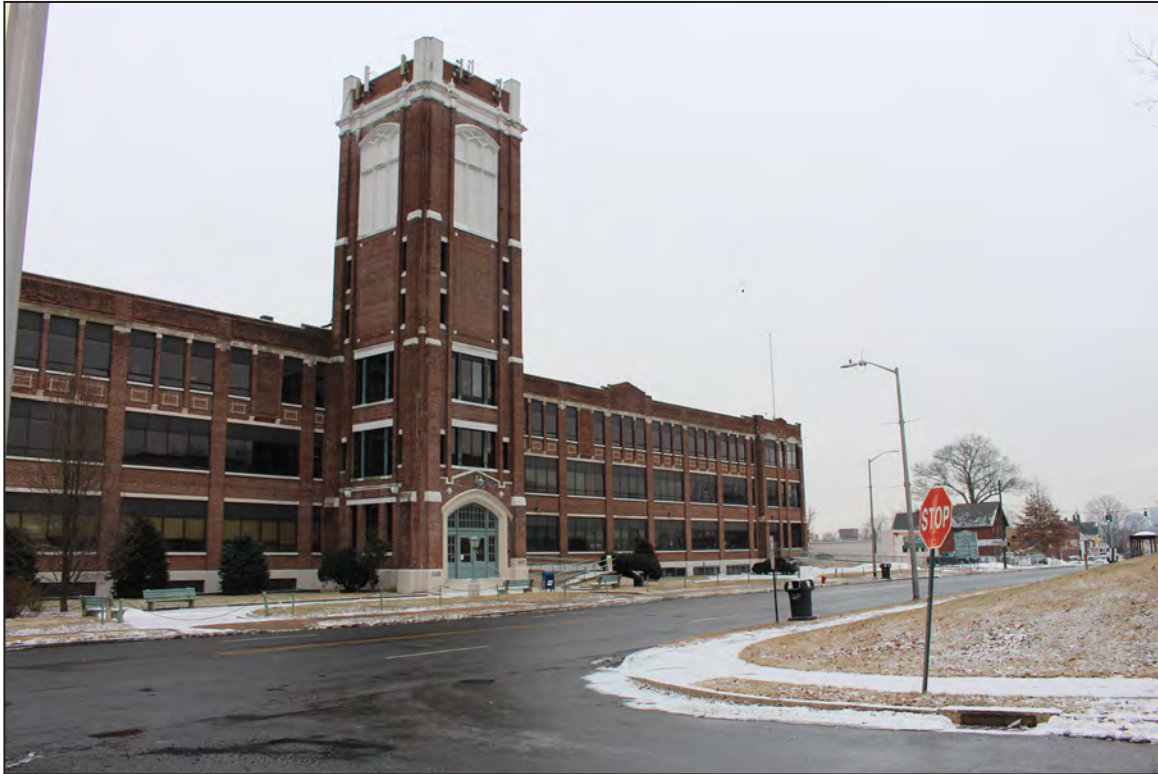
17. Main Office/Factory Building, West Elevation, looking southeast.
