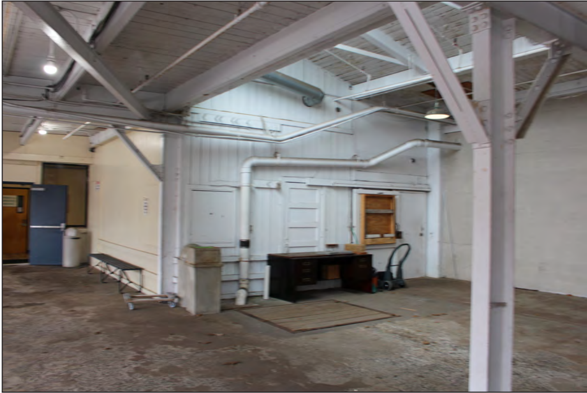
51. Main Office/Factory Building, South Elevation, looking northwest.
