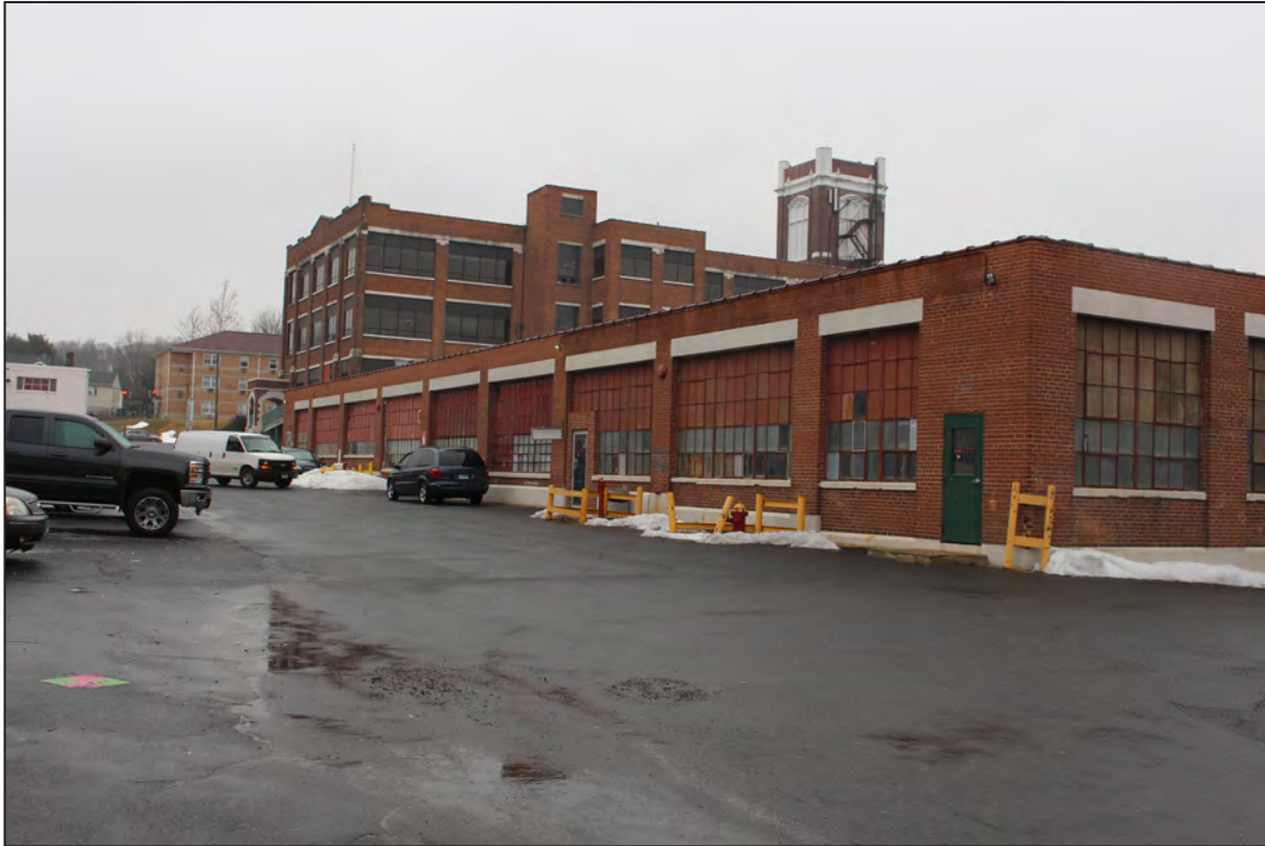
77. Site View, looking northwest. Factory/Garage Building in foreground, Main Office/Factory Building in background.
