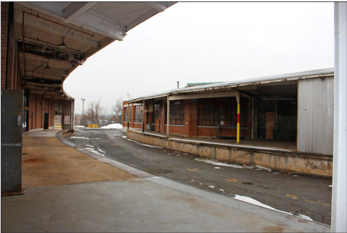
44. Site View, looking southeast. Factory/Warehouse Building (left) and Factory/Garage Building (right).
