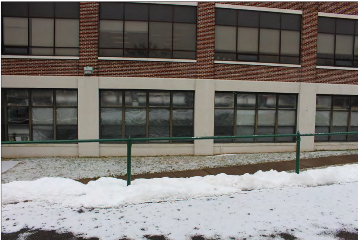
26. Main Office/Factory Building, North Elevation, looking south.
