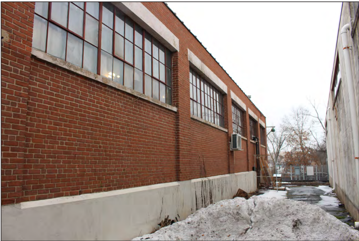
78. Factory/Garage Building, South Elevation, looking northeast.
