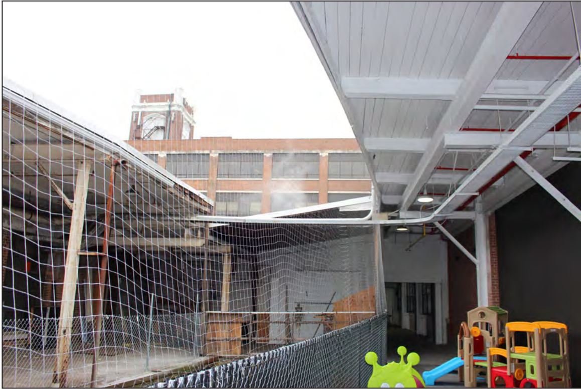
45. Site View, looking west. Main Office/Factory Building in background, Factory/Warehouse Building (right), Factory/Garage Building (left).
