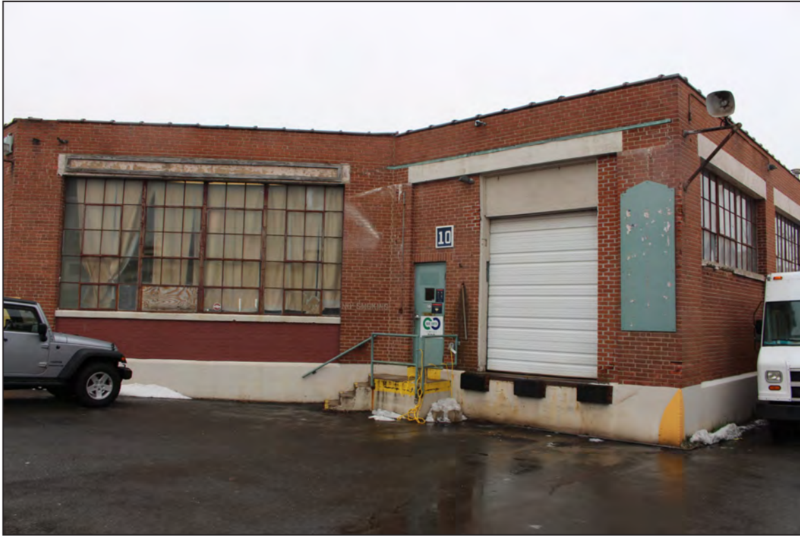
75. Factory/Garage Building, South and West Elevations, looking northeast.
