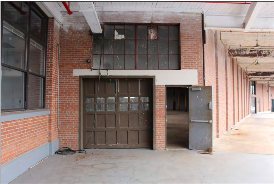
46. Factory/Warehouse Building, South Elevation, looking east.
