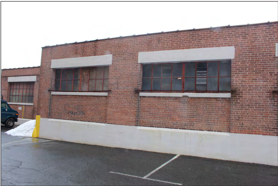
58. Factory/Garage Building, West Elevation, looking northeast.
