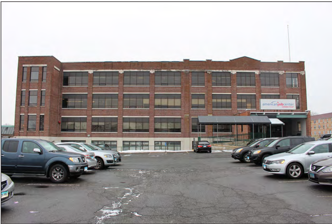
24. Main Office/Factory Building, North Elevation, looking south.
