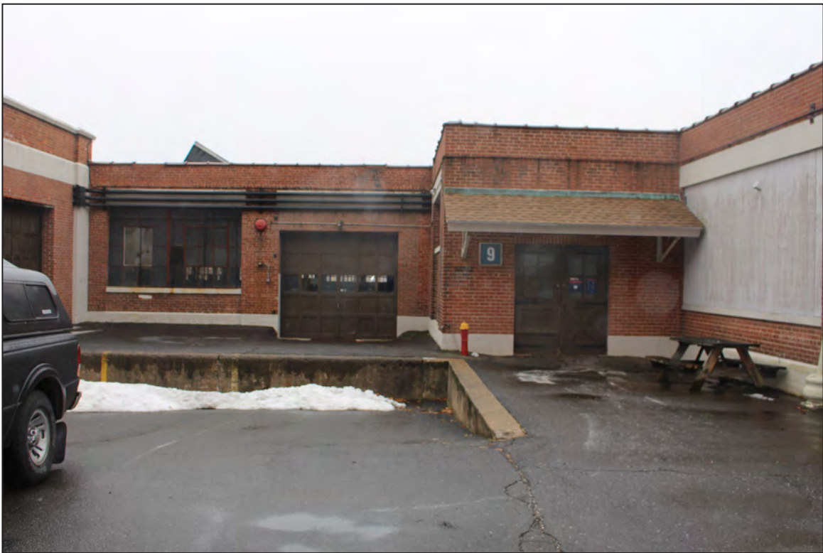
56. Factory/Garage Building, West Elevation, looking east.
