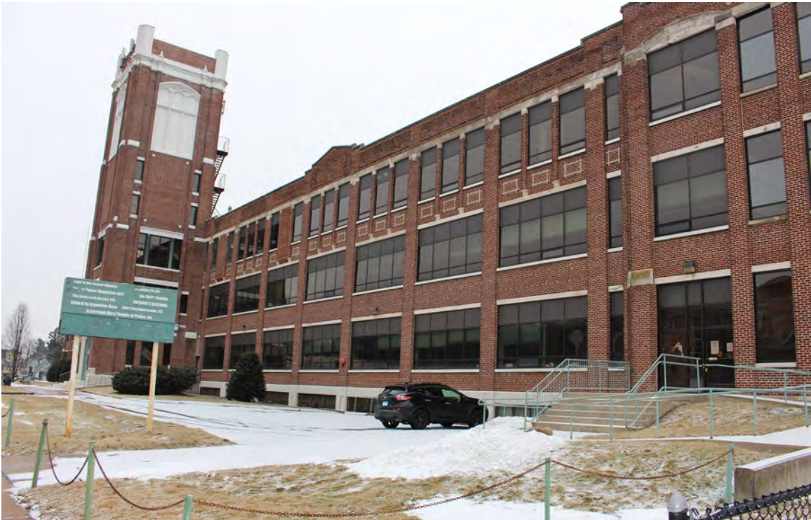
1. Main Office/Factory Building, West Elevation, looking northeast.
