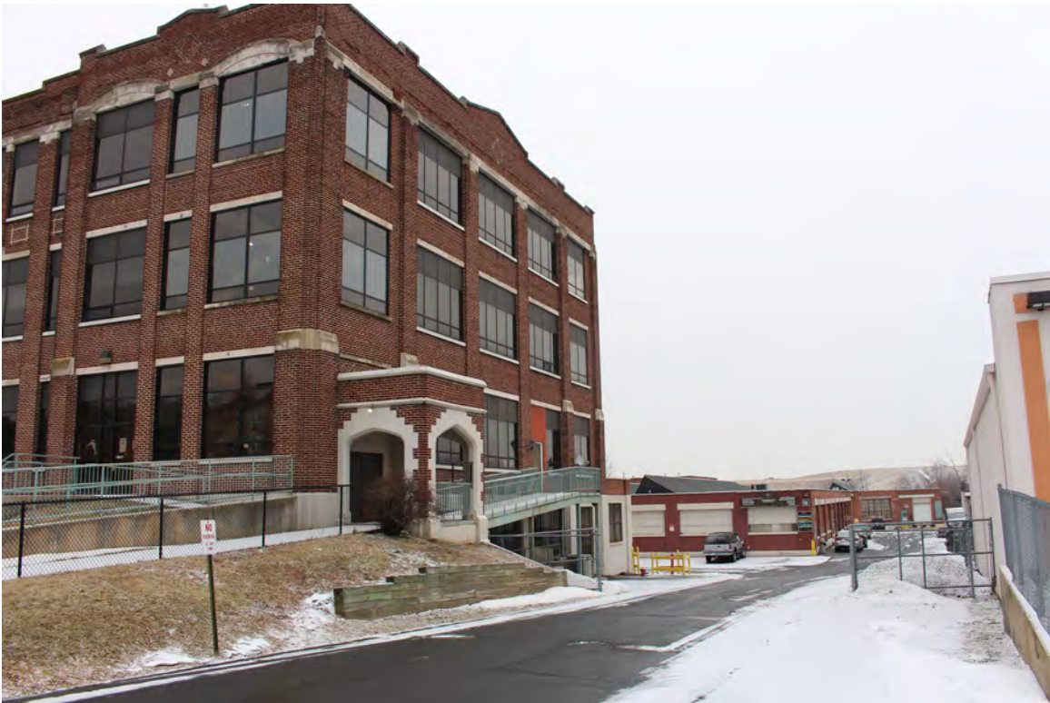
2. Main Office/Factory Building, South and West Elevations, looking northeast.
