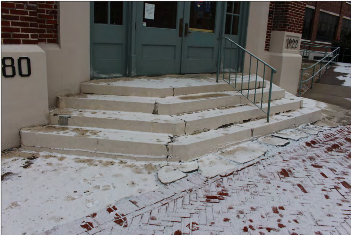
14. Main Office/Factory Building, West Elevation, looking southeast.
