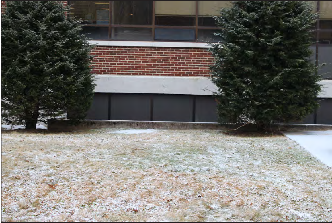
21. Main Office/Factory Building, West Elevation, looking east.
