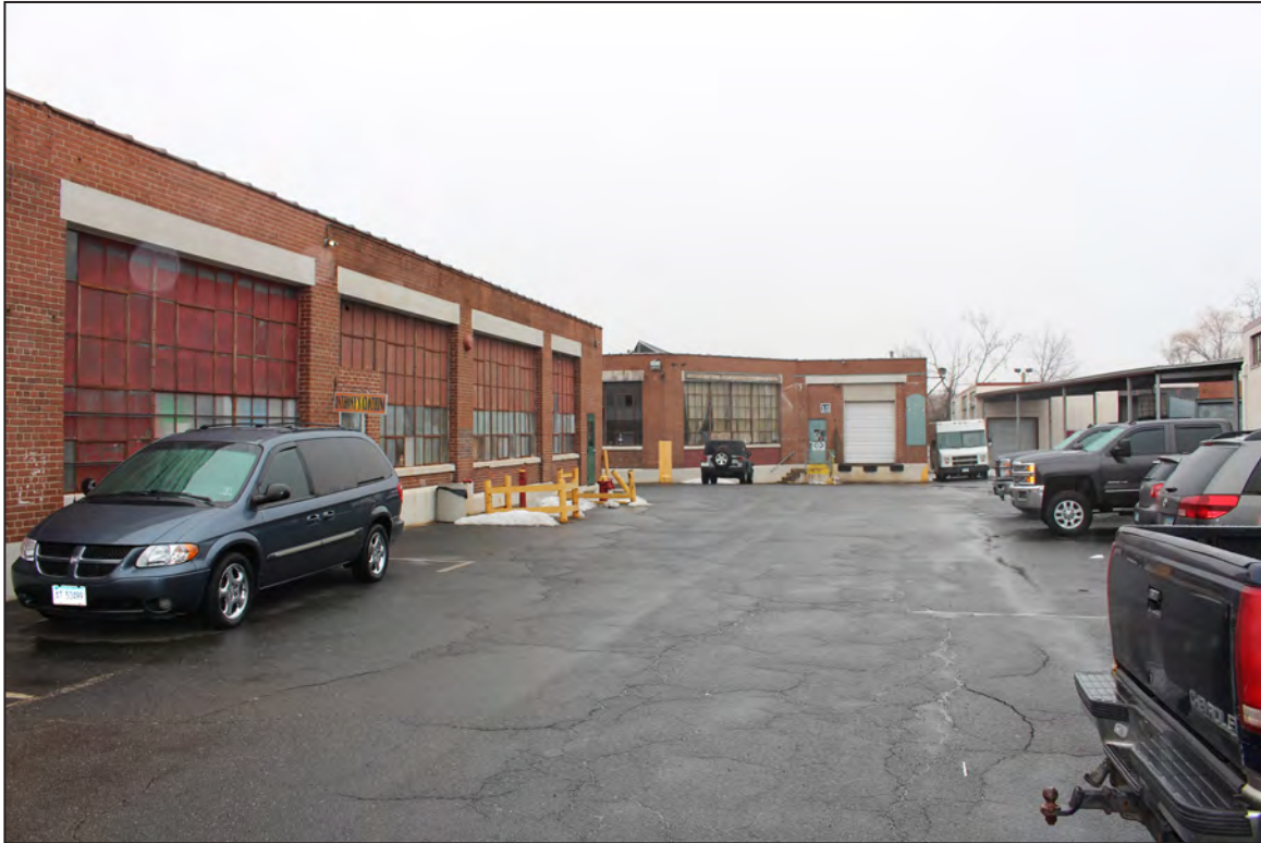
69. Site View, looking east. Factory/Garage Building to the left.
