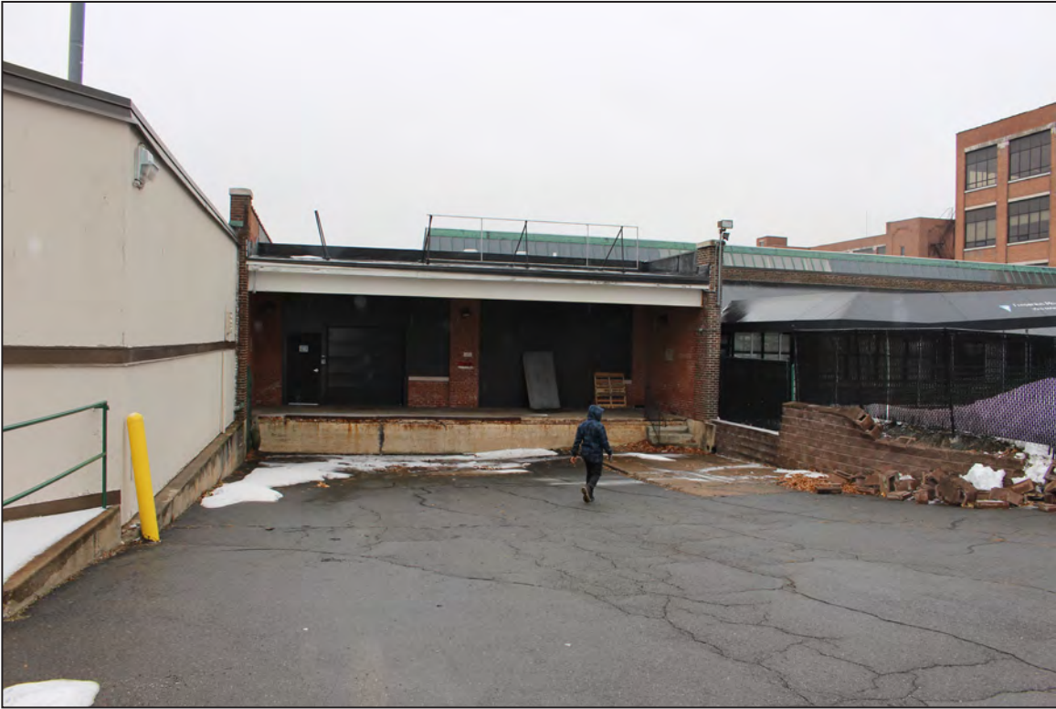
31. Factory/Warehouse Building, North Elevation, looking south.
