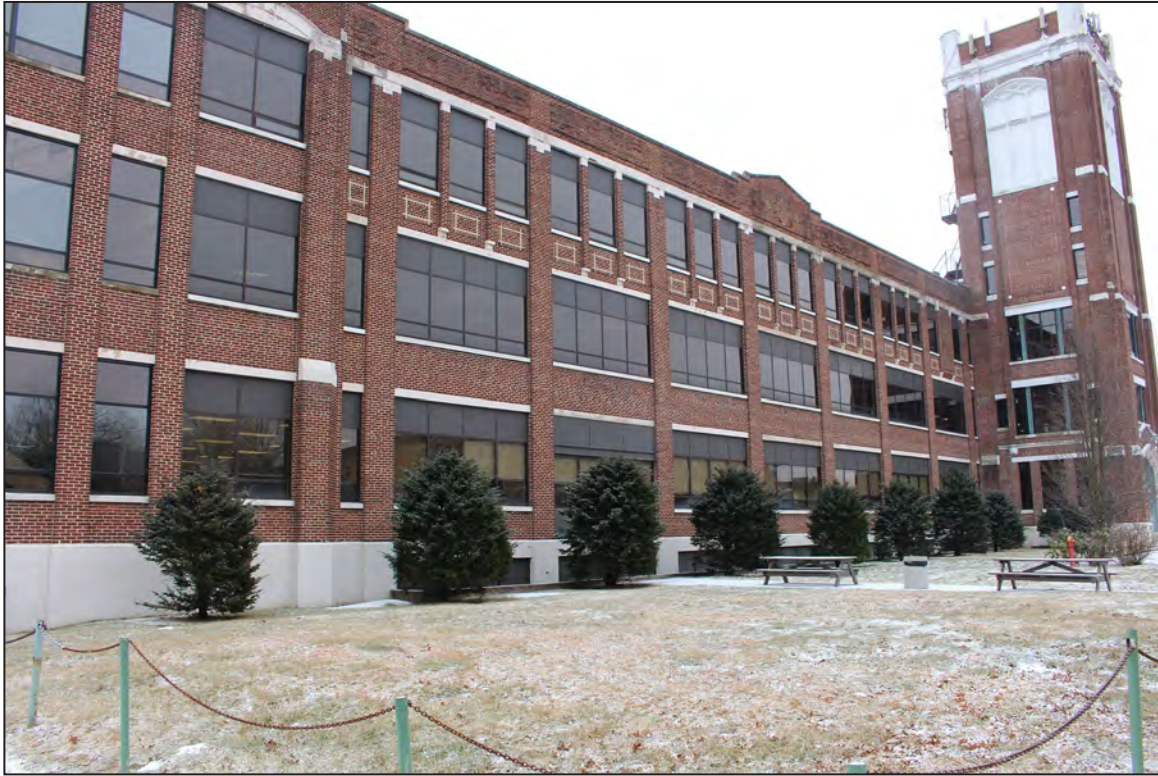
19. Main Office/Factory Building, West Elevation, looking southeast.
