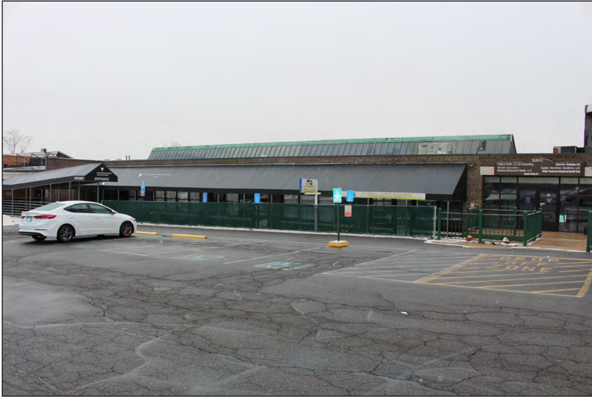
29. Factory/Warehouse Building, North Elevation, looking southeast.
