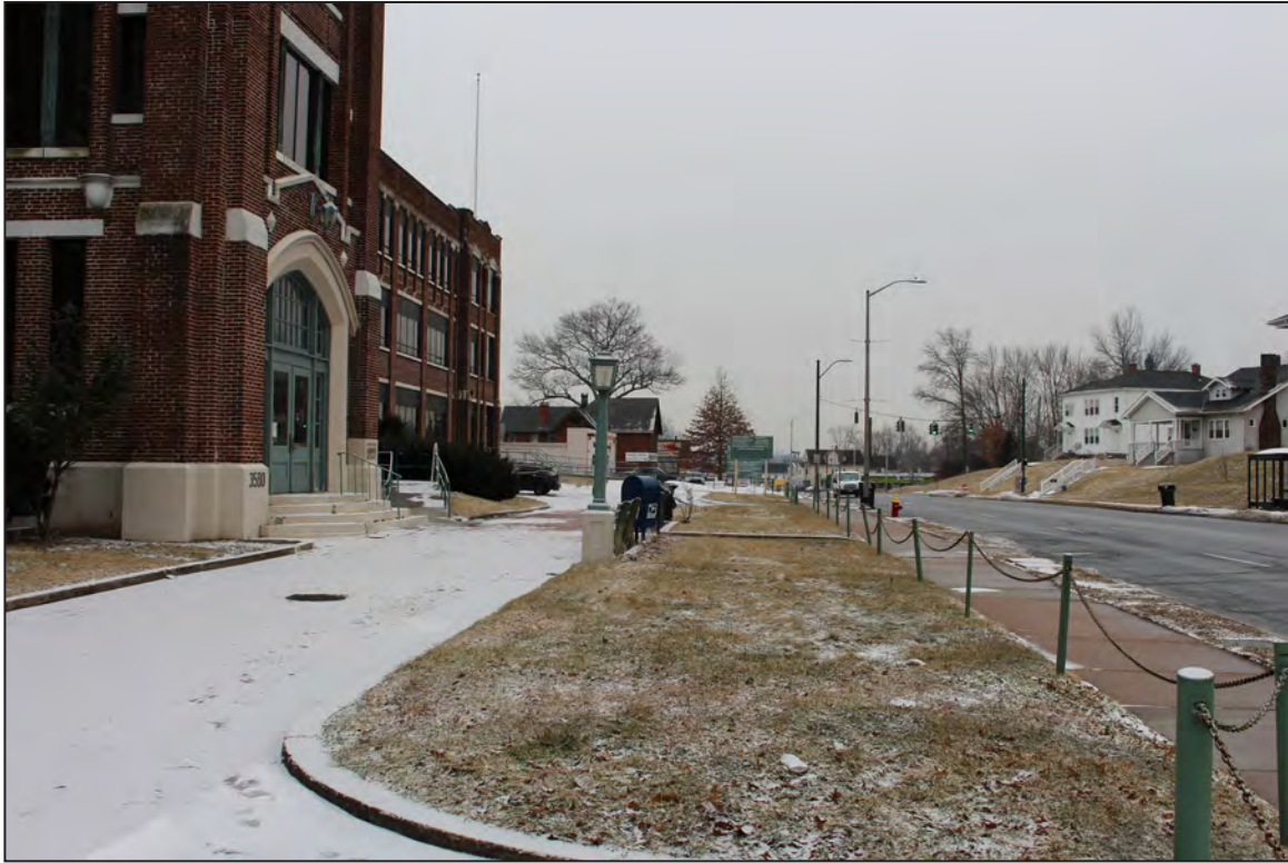
15. Main Office/Factory Building, West Elevation, looking south.
