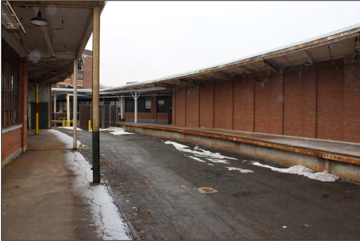
41. Factory/Warehouse Building, South Elevation, looking northwest.
