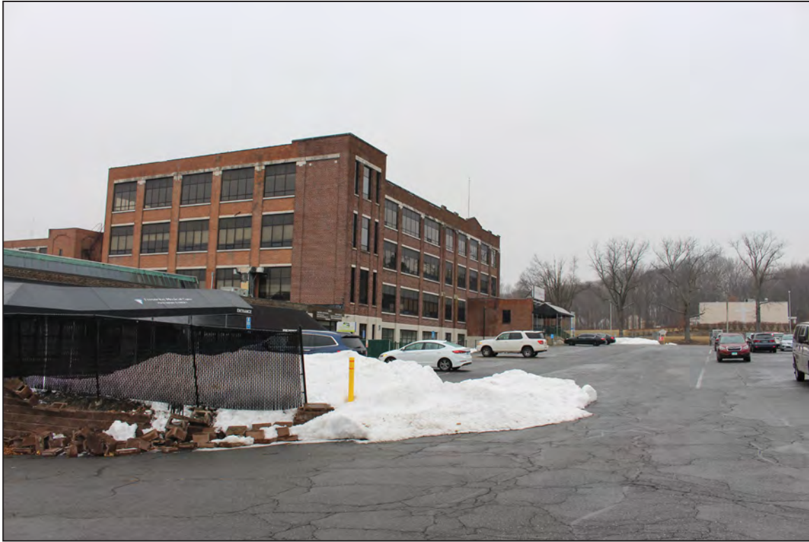
33. Main Office/Factory Building, North and East Elevations, looking southwest.
