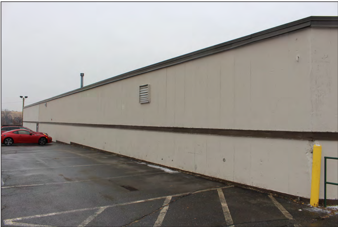
34. Factory/Warehouse Building, North Elevation, looking southeast.
