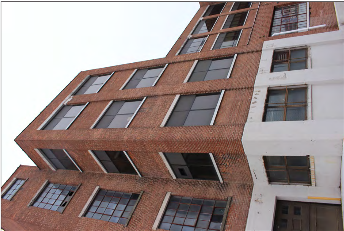
64. Main Office/Factory Building, East Elevation, looking northwest.
