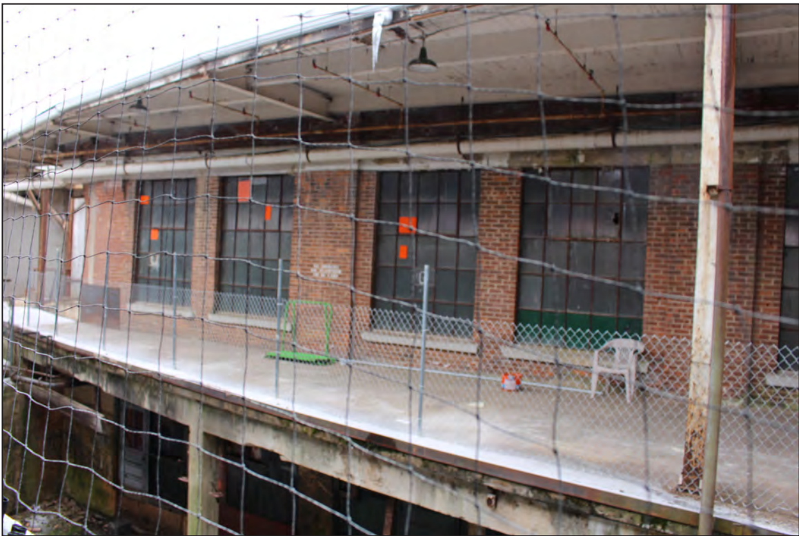
48. Factory/Garage Building, North Elevation, looking south.
