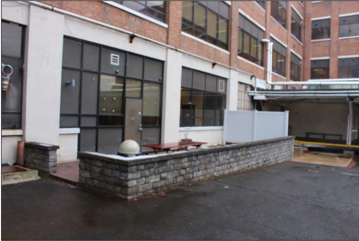
53. Main Office/Factory Building, East Elevation, looking northwest.
