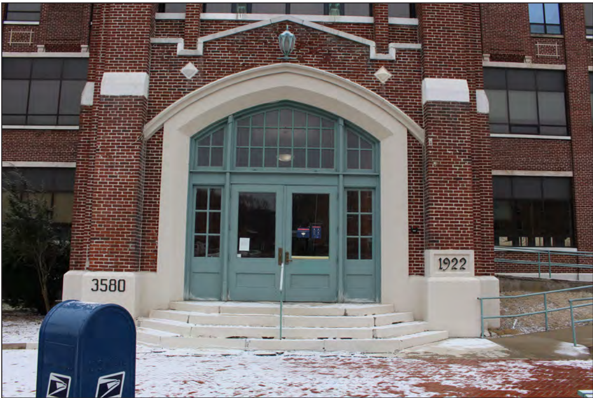
12. Main Office/Factory Building, West Elevation, looking east.
