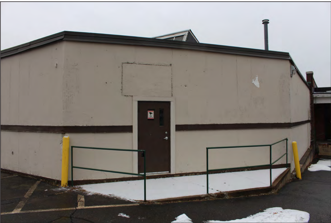
32. Factory/Warehouse Building, North Elevation, looking southeast.
