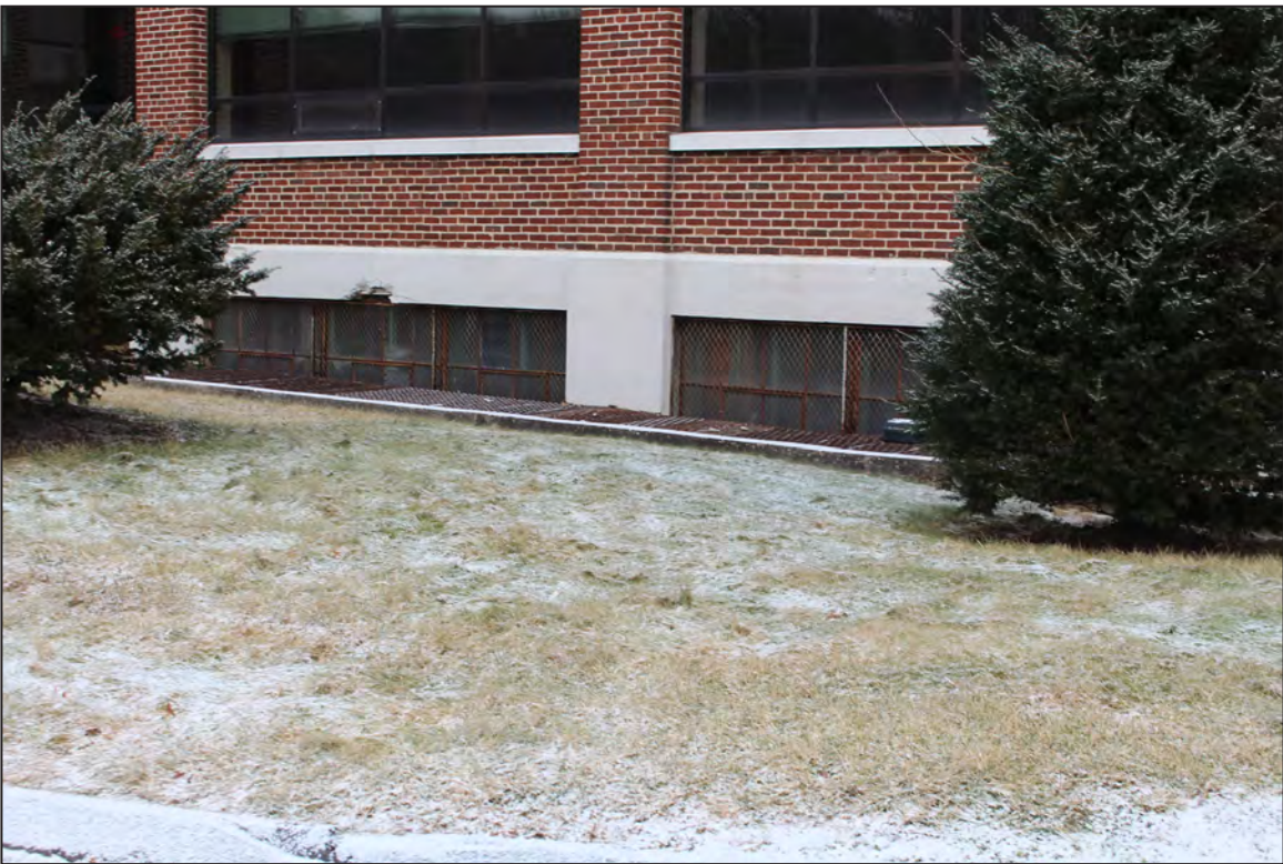
10. Main Office/Factory Building, West Elevation, looking northeast.
