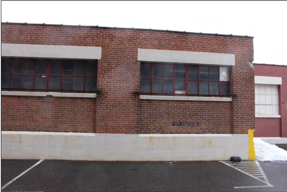
59. Factory/Garage Building, West Elevation, looking east.
