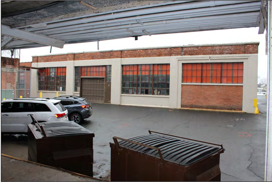
49. Factory/Garage Building, looking south.
