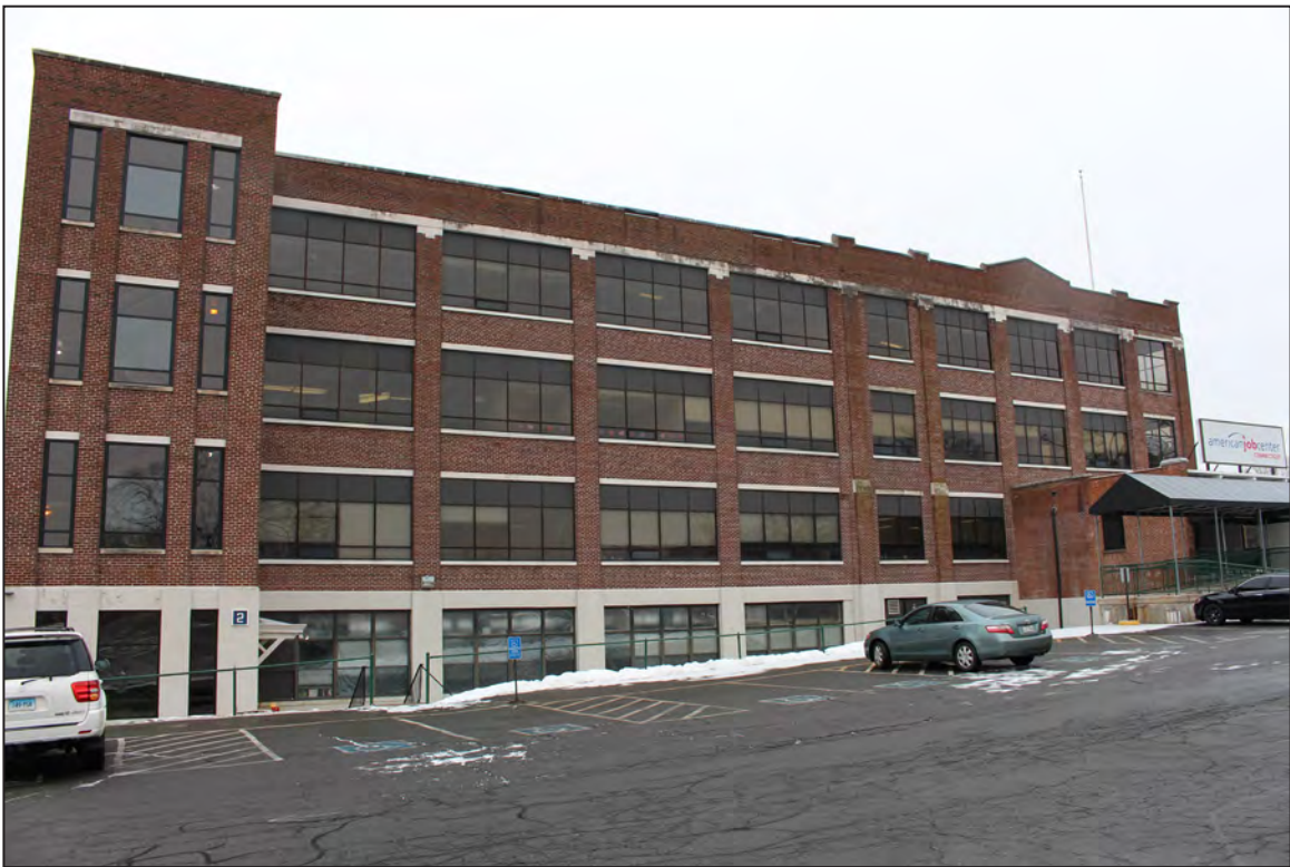
28. Main Office/Factory Building, North Elevation, looking southwest.
