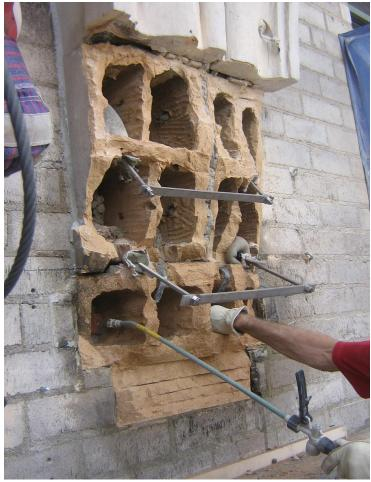
Custom SYSTEM 45 using RL-2 form and pour application at 230 Park Ave, NYC. Anchor system installed into Terra Cotta.
