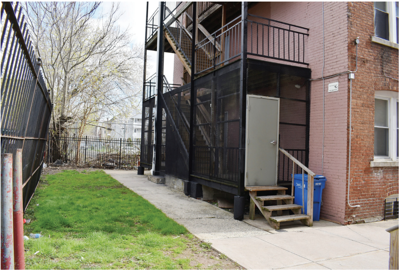
5. Rear (west) elevation and yard
