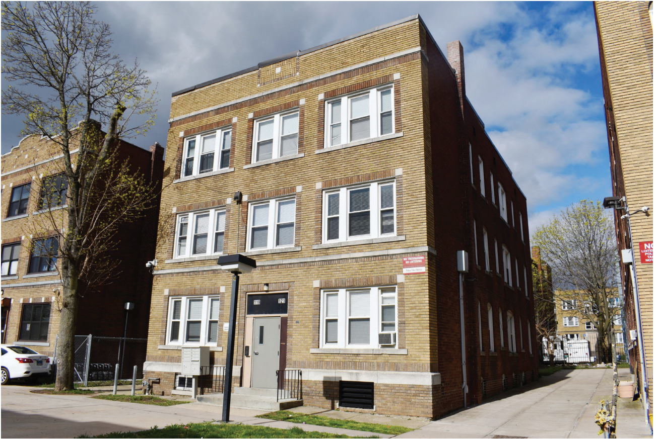
3. Façade (east) and side (north) elevations
