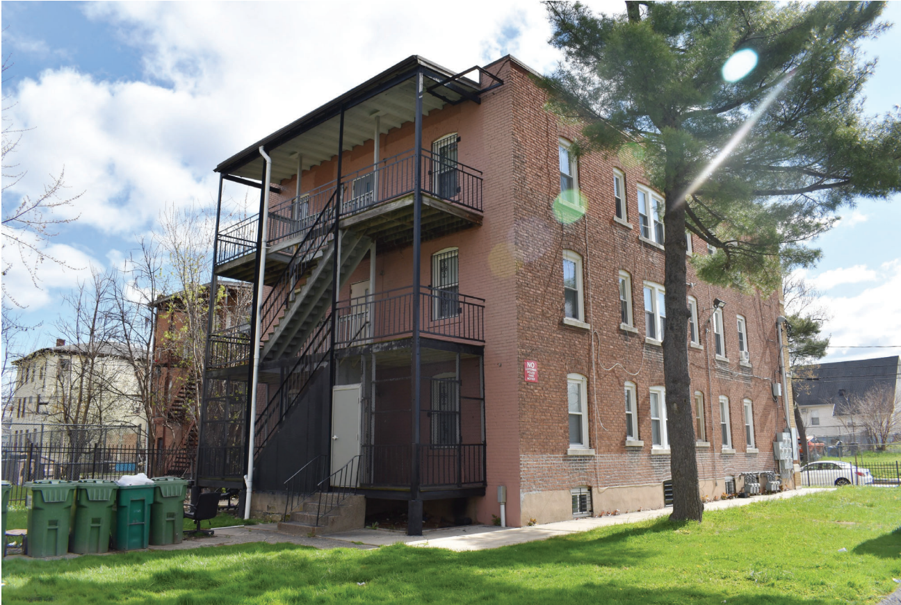
4. Side (south) and rear (west) elevations
