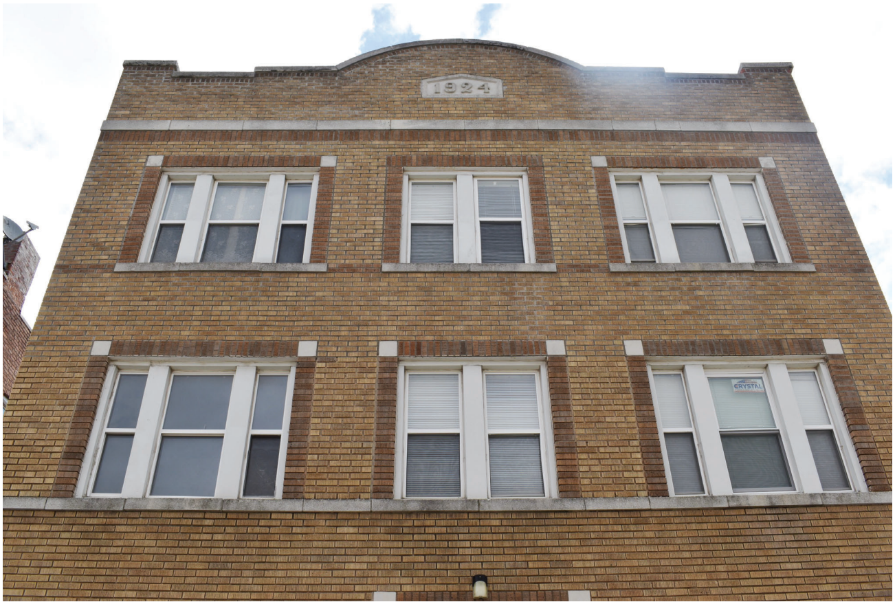
3. Façade (west) elevation
