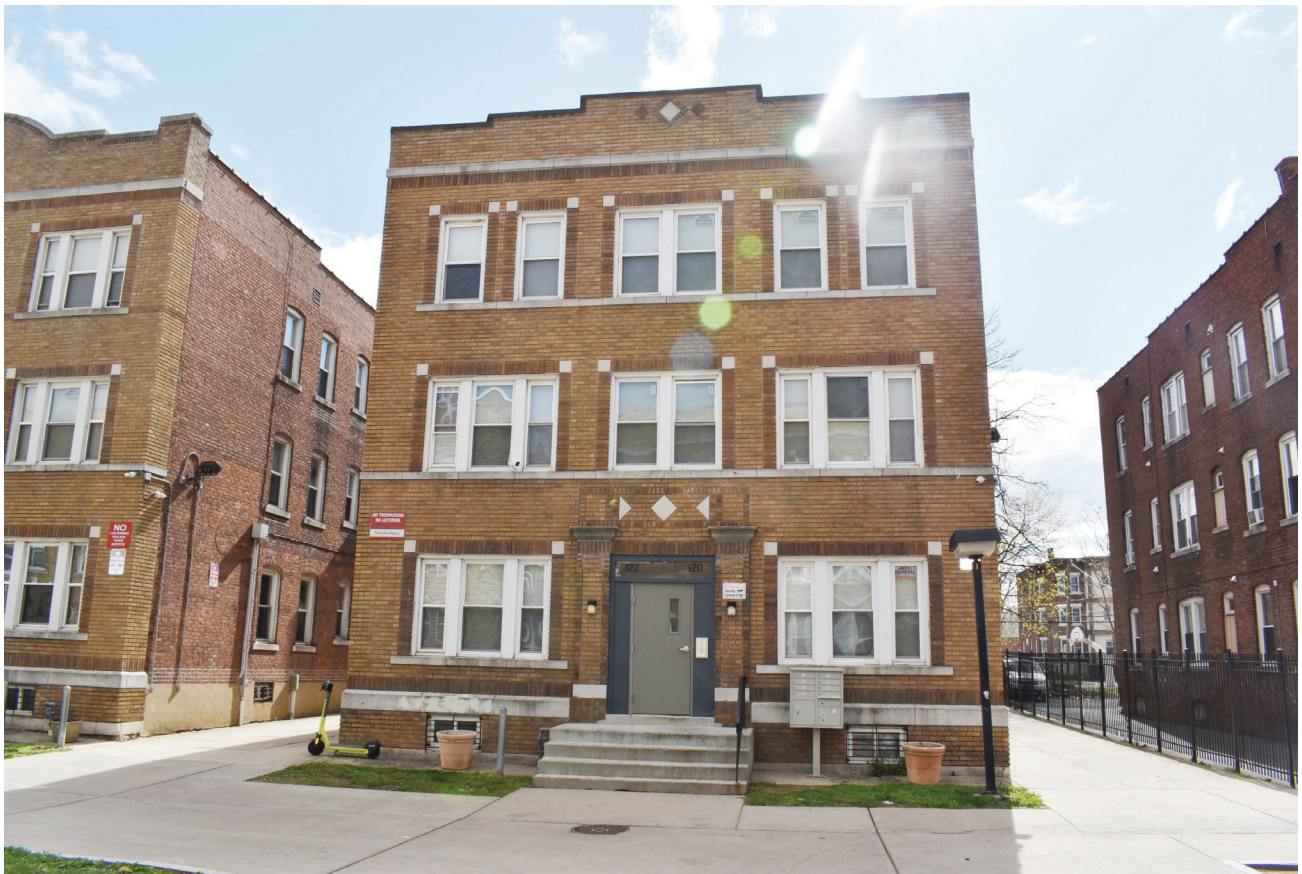
1. Façade (west) elevation
