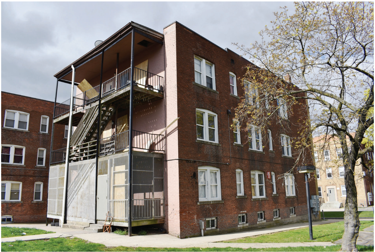
5. Rear (east) and side (north) elevations
