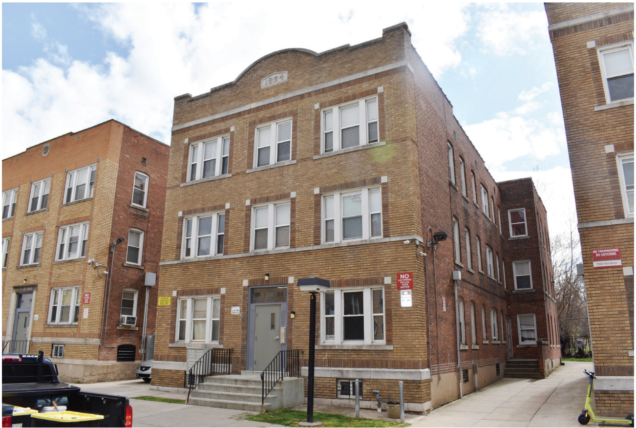
9. Side (south) and façade (west) elevations
