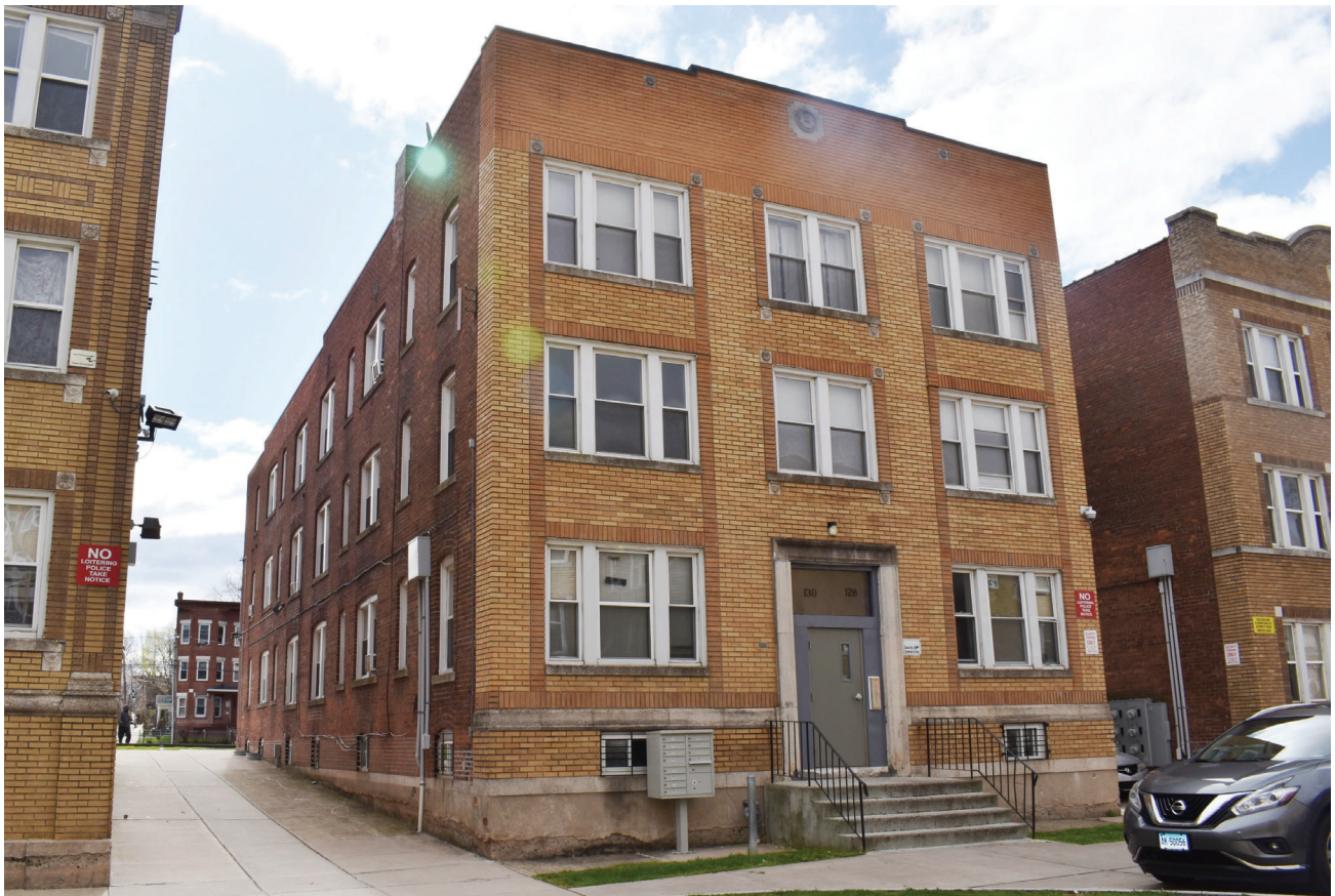
1. Façade (west) elevation
