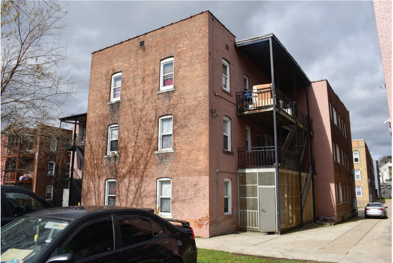
6. Rear (east) and side (north) elevations
