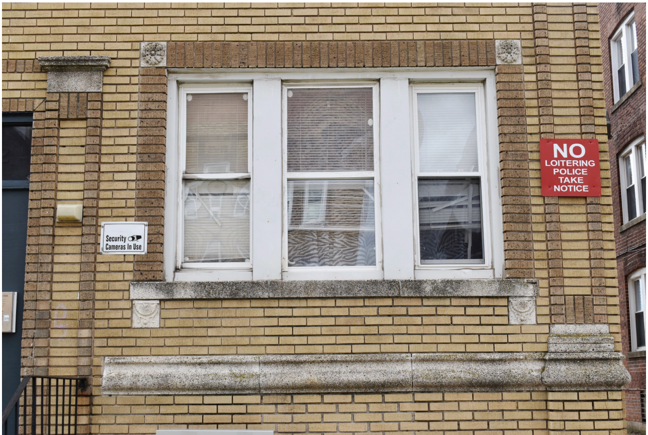
3. Façade (west) elevation, window detail
