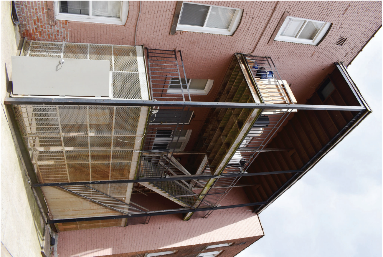
5. Side (north) elevation, deck detail
