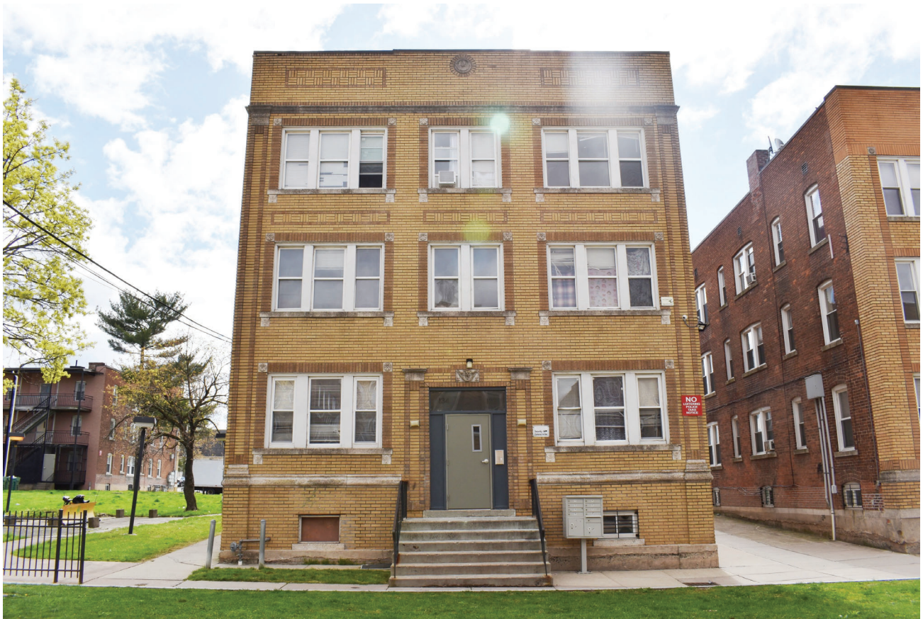
1. Façade (west) elevation
