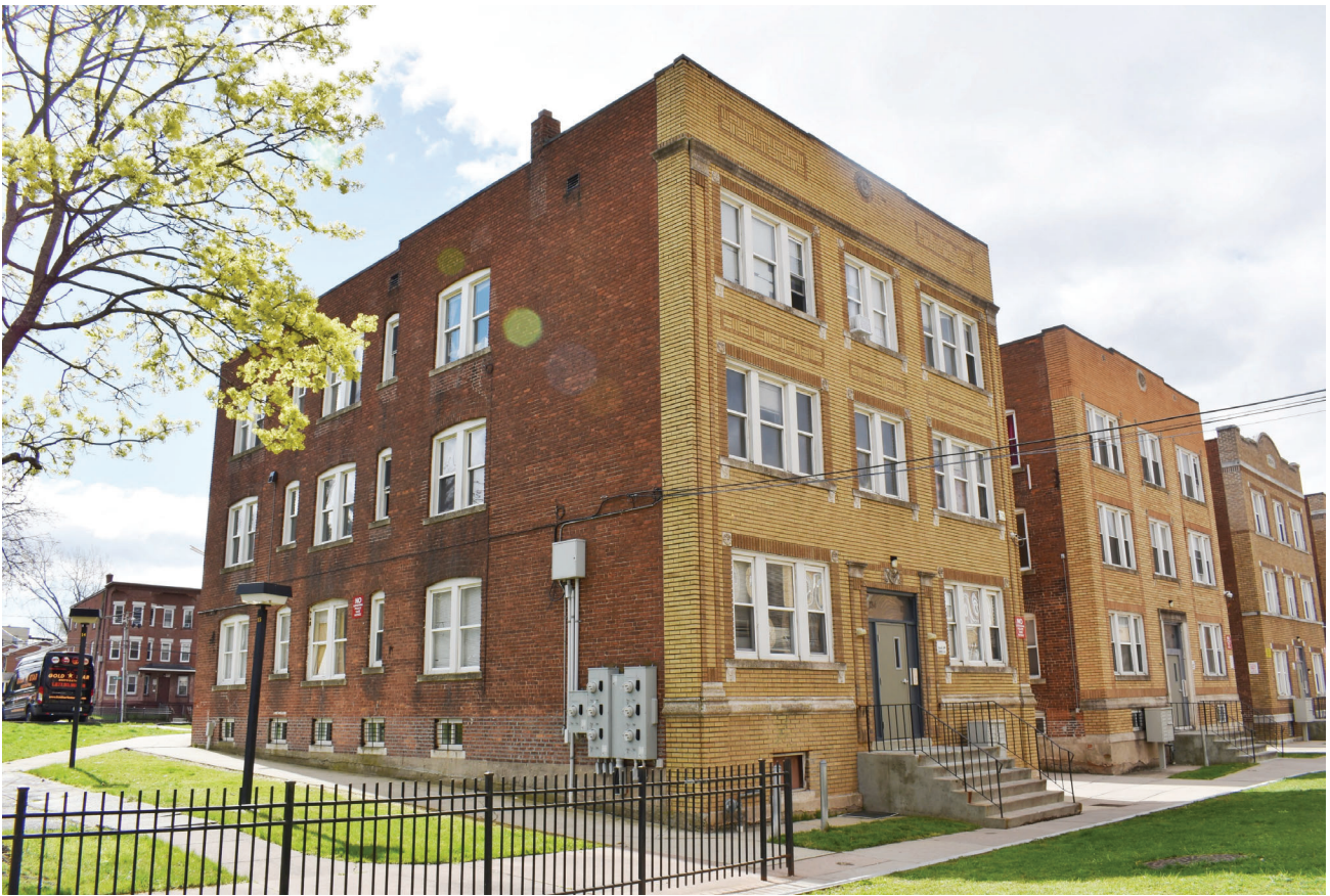
7. Façade (west) and side (north) elevations
