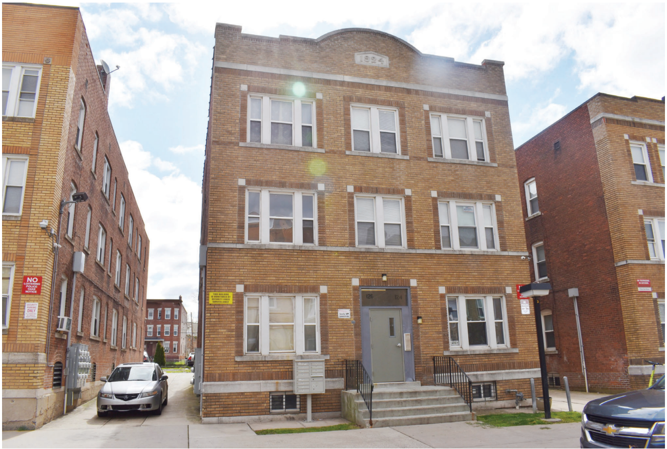
1. Façade (west) elevation
