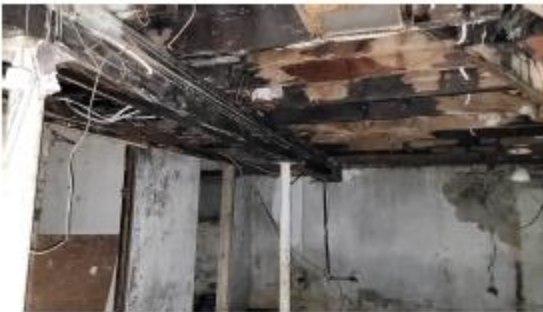
5. Basement and 1 st floor framing at front.
