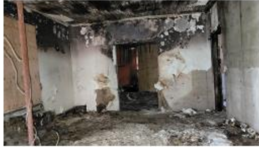
10. 2 nd floor, west side.
