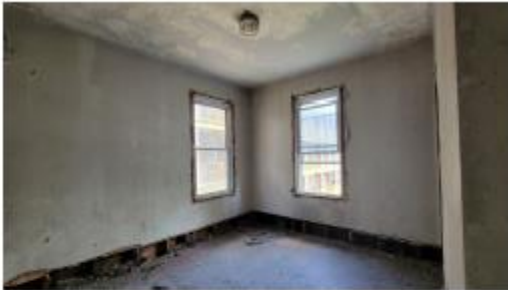
13. 2 nd floor, southeast corner.
