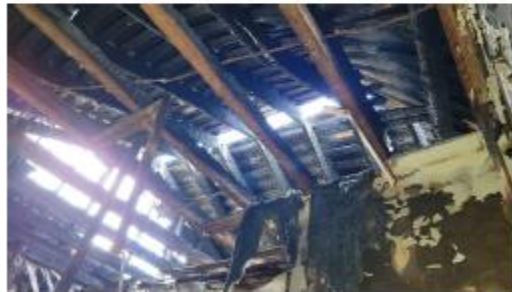
16. Roof and attic floor framing front.
