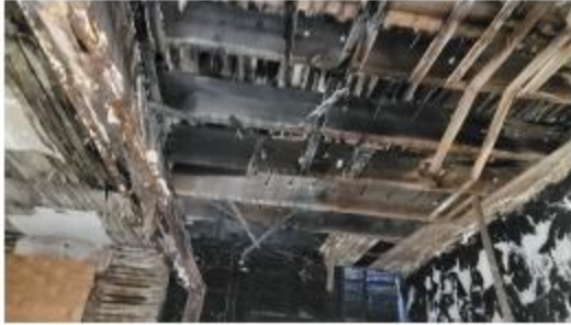
9. Second floor framing at front.
