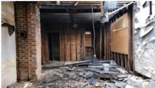
15. 3 rd floor, west side looking south.
