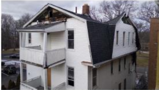
3. Rear and east side.
