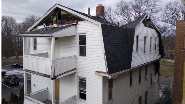
3. Rear and east side.
