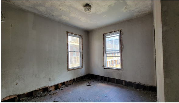
13. 2 nd floor, southeast corner.
