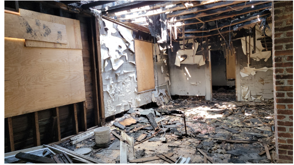
14. 3 rd floor, west side.
