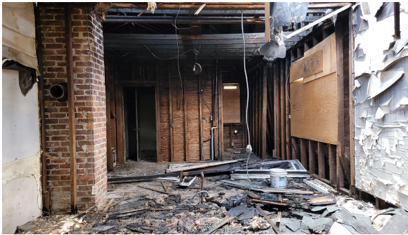
15. 3 rd floor, west side looking south.
