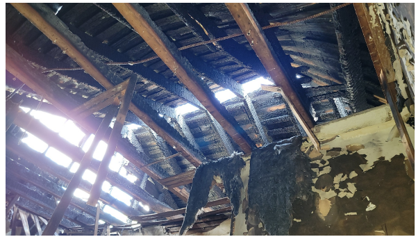
16. Roof and attic floor framing front.
