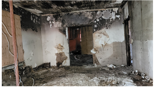
10. 2 nd floor, west side.
