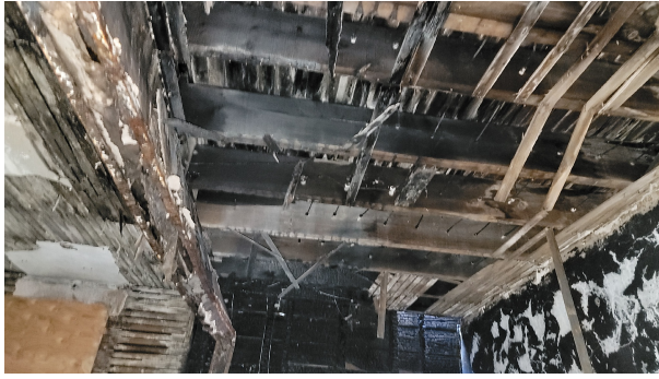
9. Second floor framing at front.
