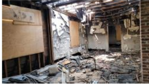
14. 3 rd floor, west side.
