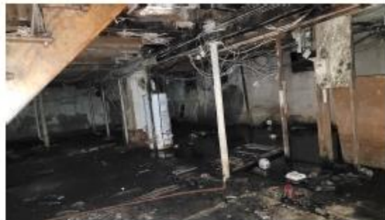
6. Basement looking toward rear.
