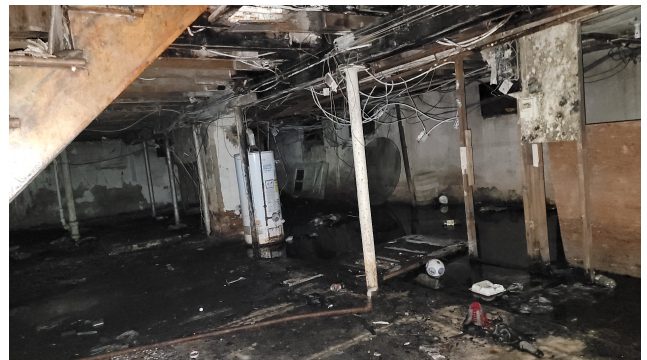
6. Basement looking toward rear.
