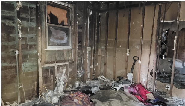
7. 1st floor southwest corner
