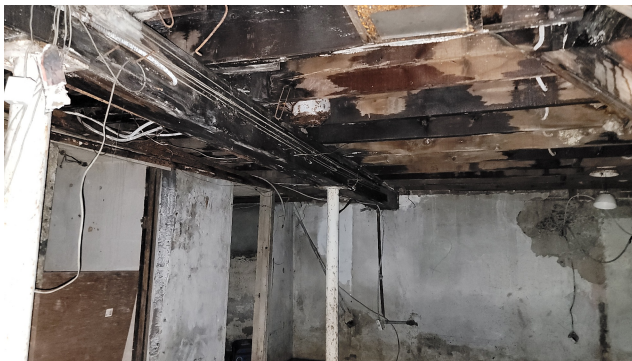
5. Basement and 1 st floor framing at front.
