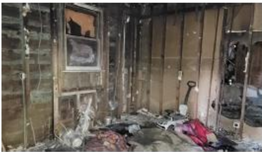
7. 1st floor southwest corner
