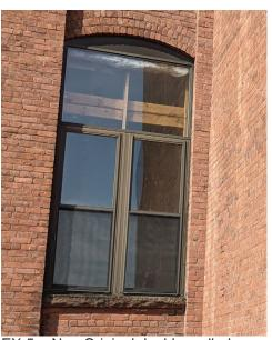
EX-5 - Non-Original double mulled double hung aluminum window with arched transom. No exterior caulking is visible at the aluminum replacement windows
