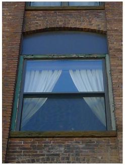
EX-8- Replacement aluminum double hung window with carpentry in fill above
