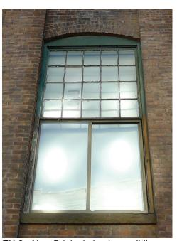
EX-3 - Non-Original aluminum sliding window installed under original 20 pane upper sash
