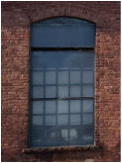
EX-2 - Original 20/20 double hung arched metal window with wire glass
