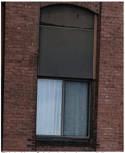
EX-4- Non-Original aluminum sliding window installed under original 20 pane upper sash covered with plywood
