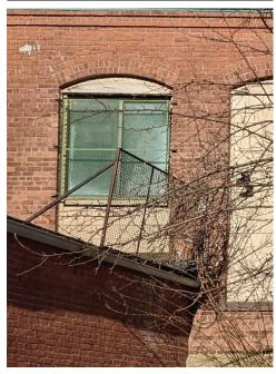
EX-19 - Replacement sliding window over masonry in fill
