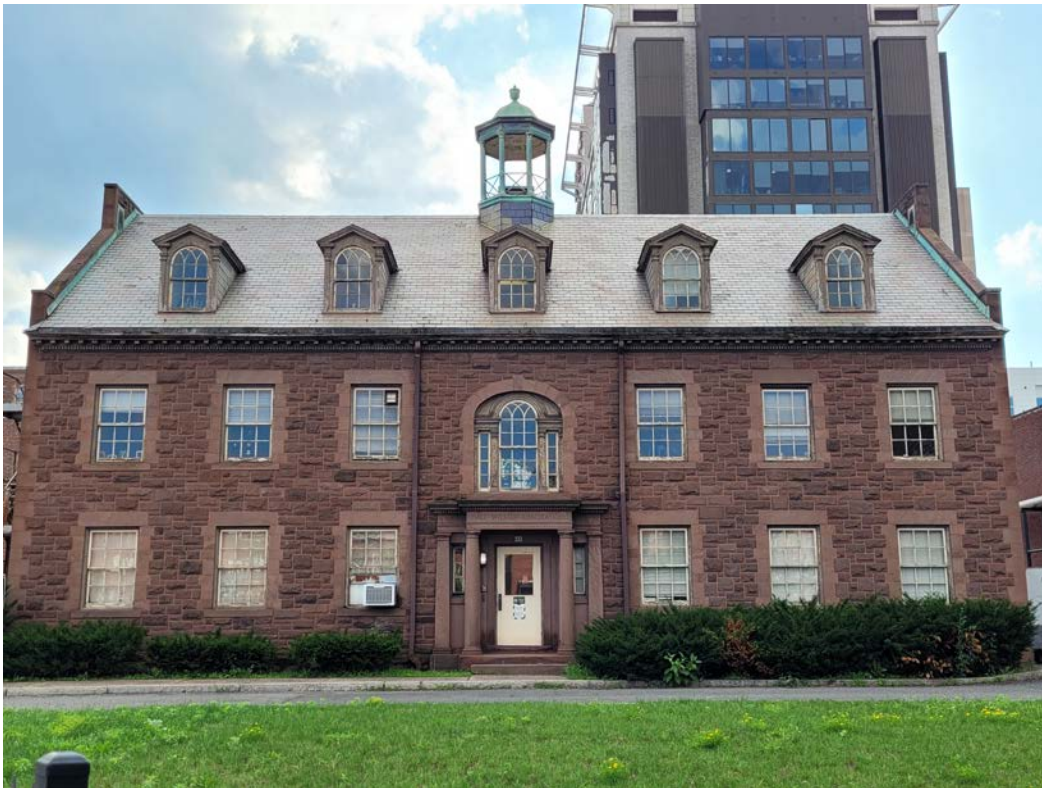
Figure 4. View of soon to be demolished Hall-Wilson Laboratory – Hartford Staff 2021
