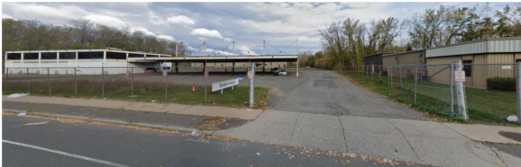
Figure 3. View of the subject property from the entrance on Elliott Street – Google Maps 2022
