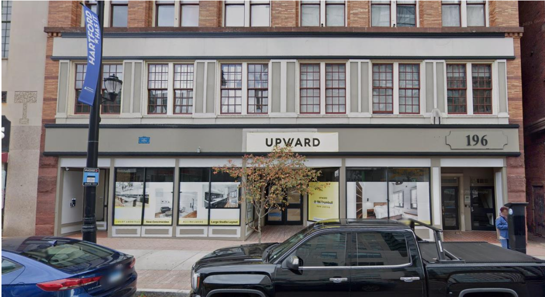
Figure 2. View of the subject property from Trumbull Street – Google Maps 2022
