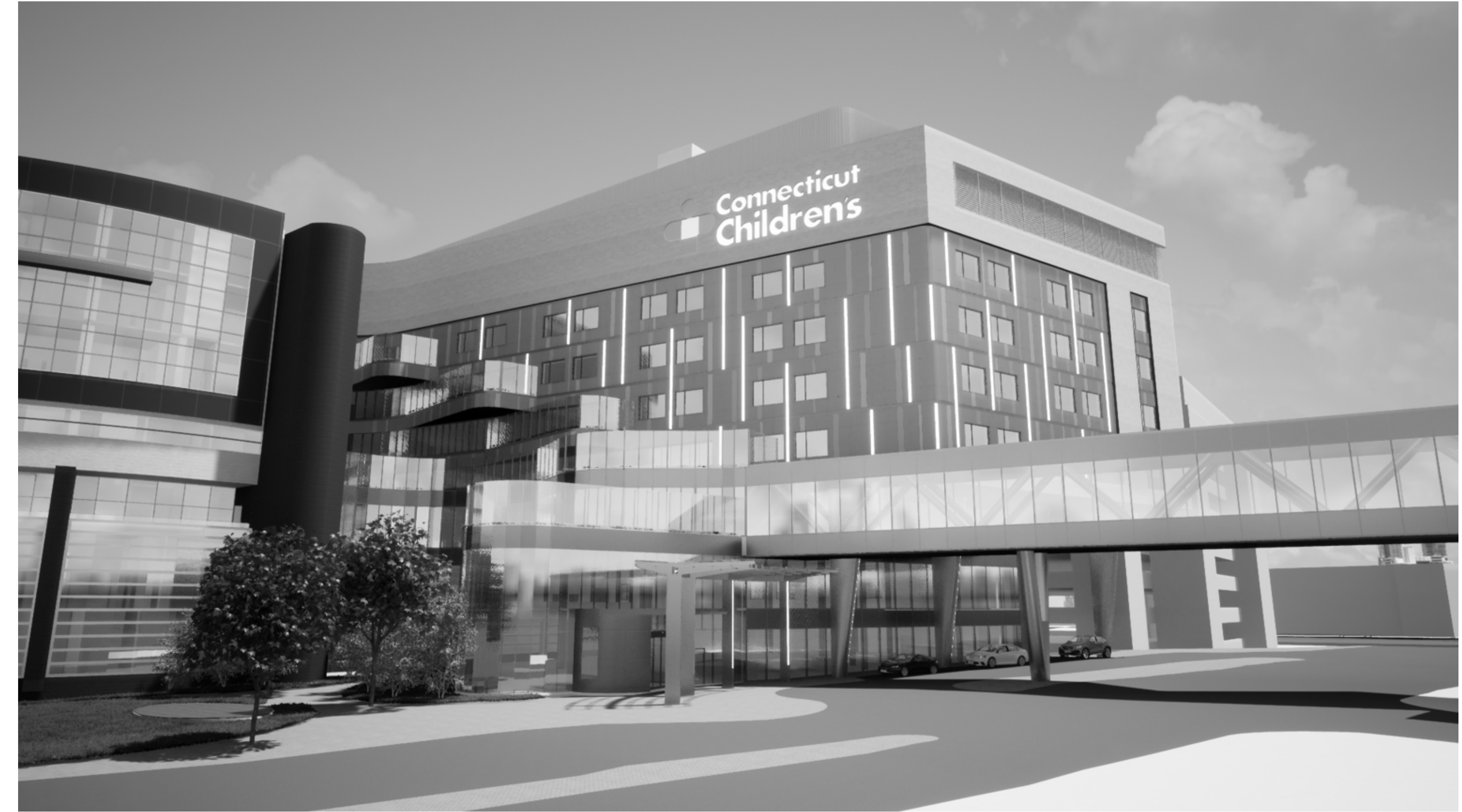
VIEW ACROSS WASHINGTON STREET LOOKING SOUTHEAST AT THE NEW TOWER EXPANSION
