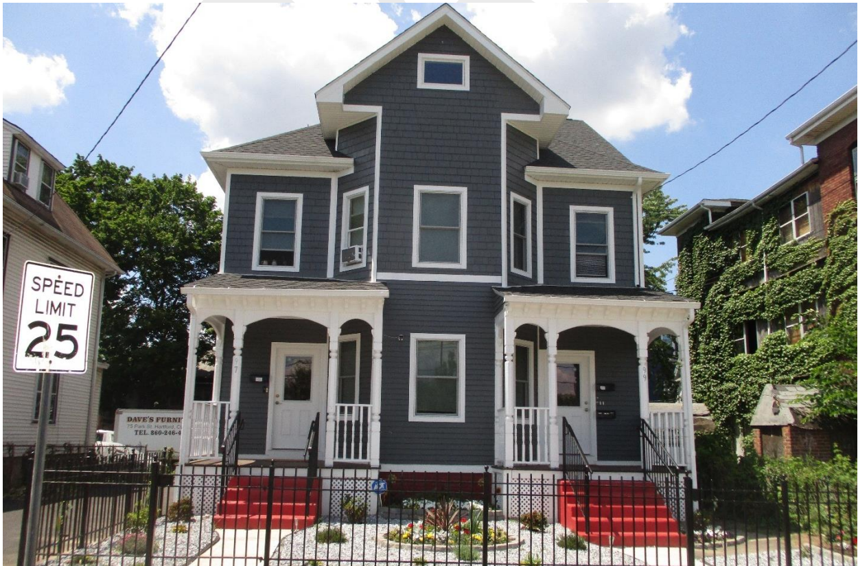
Photo: 97 Williams Street, before (top photo) and after (bottom photo). Photo citation: City of Hartford Housing Division.
