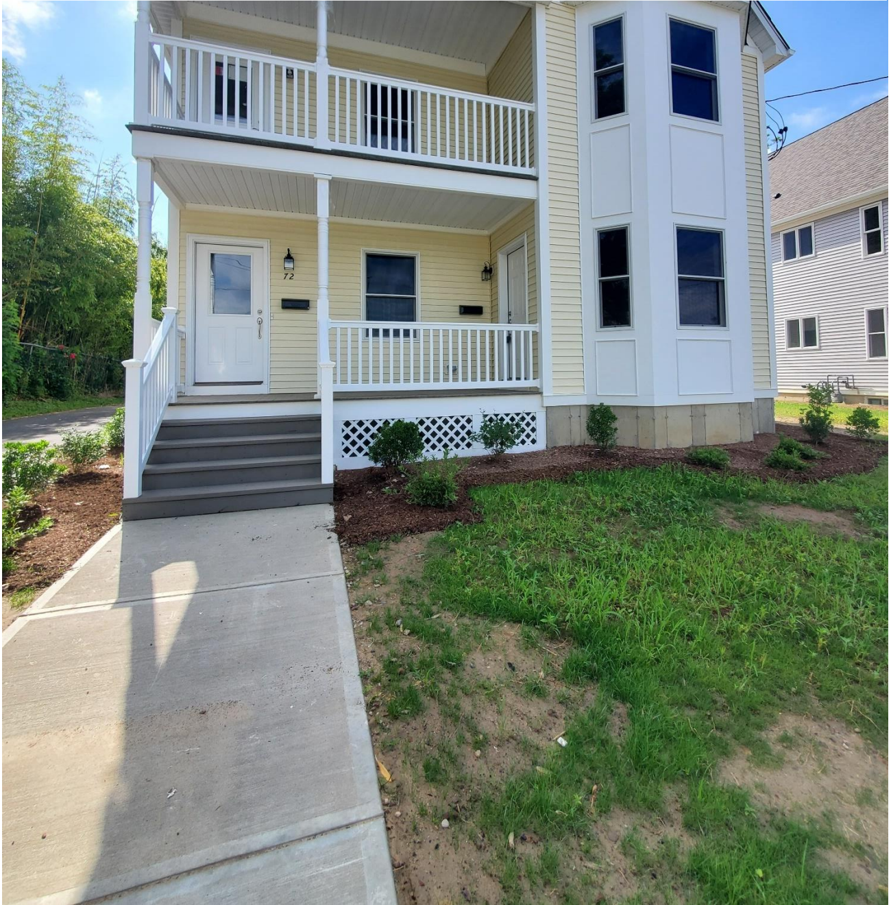
Photo: Edward Street Homeownership Opportunity. Citation: City of Hartford Housing Division.
