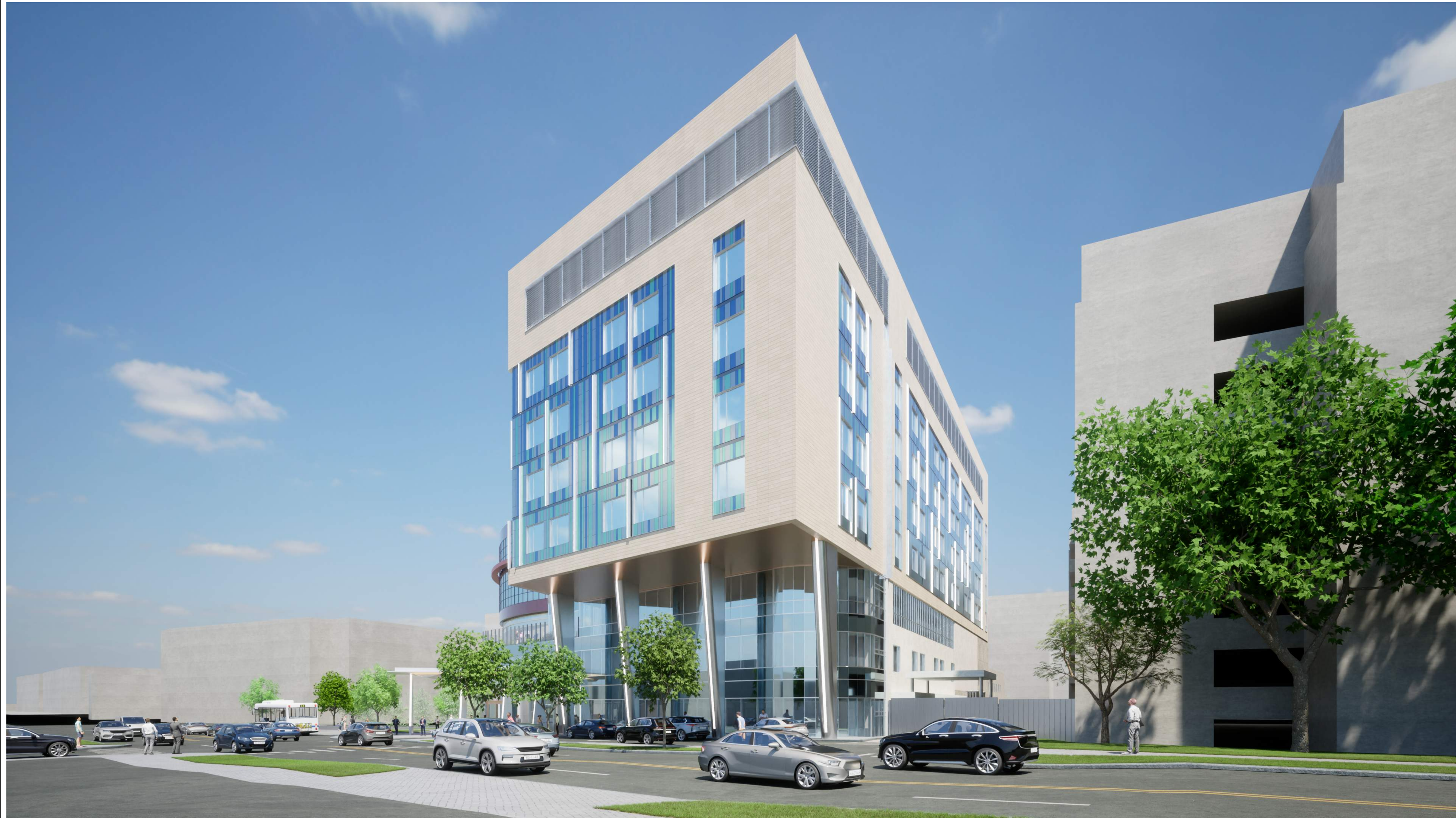
VIEW ACROSS WASHINGTON STREET LOOKING NORTHEAST AT THE NEW TOWER EXPANSION
