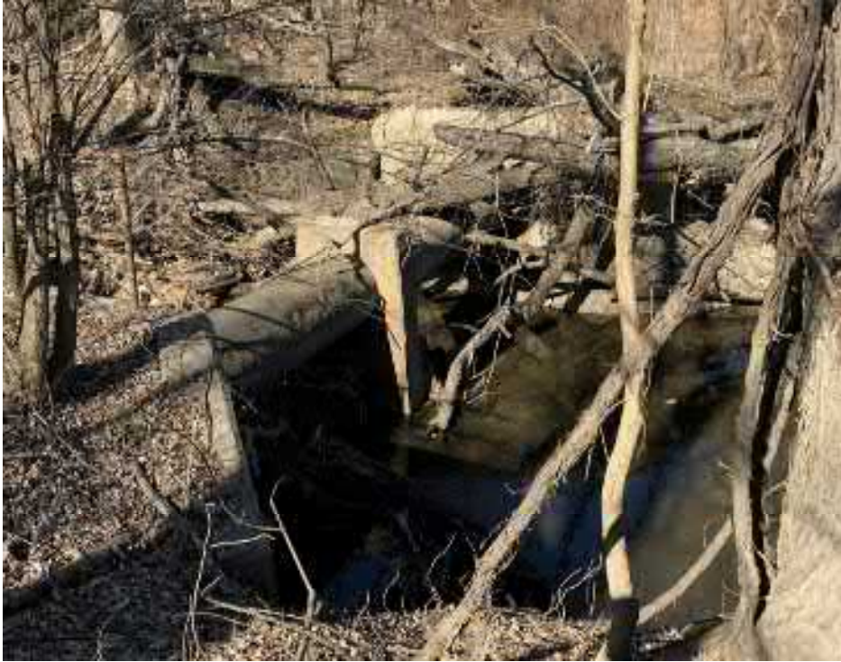
Figure 9. Utility pipe crossing Deckers Brook. Looking north.
