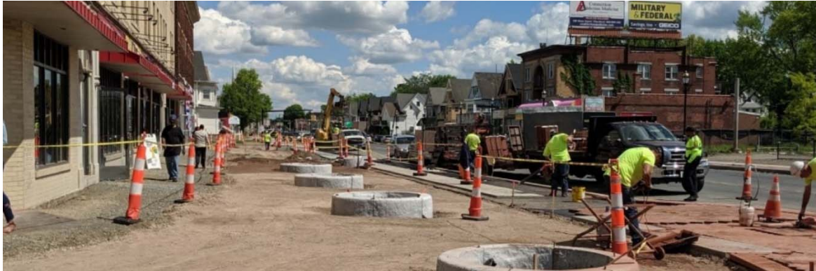
Albany Ave Street Improvement
