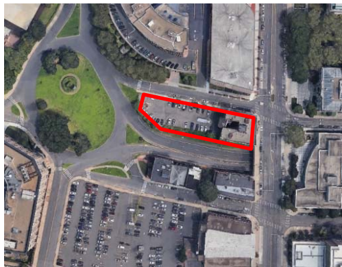
Cornerstone Building Site
