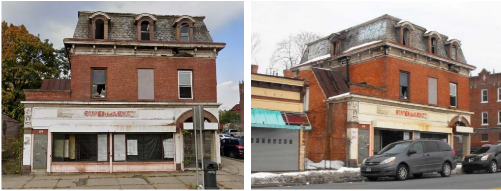
Existing 270 Albany Ave Building
