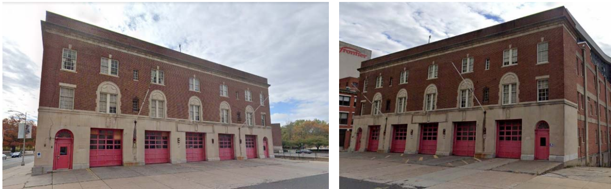
Existing Fire Headquarter Building
