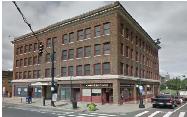
Existing Cornerstone Building
