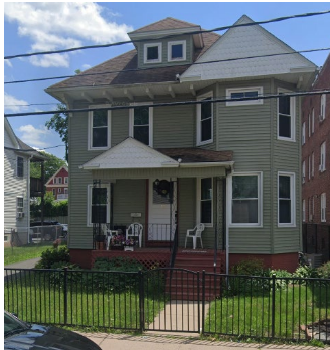
Figure 5. Existing Conditions- 17 Lincoln (Google Maps June 2021)
