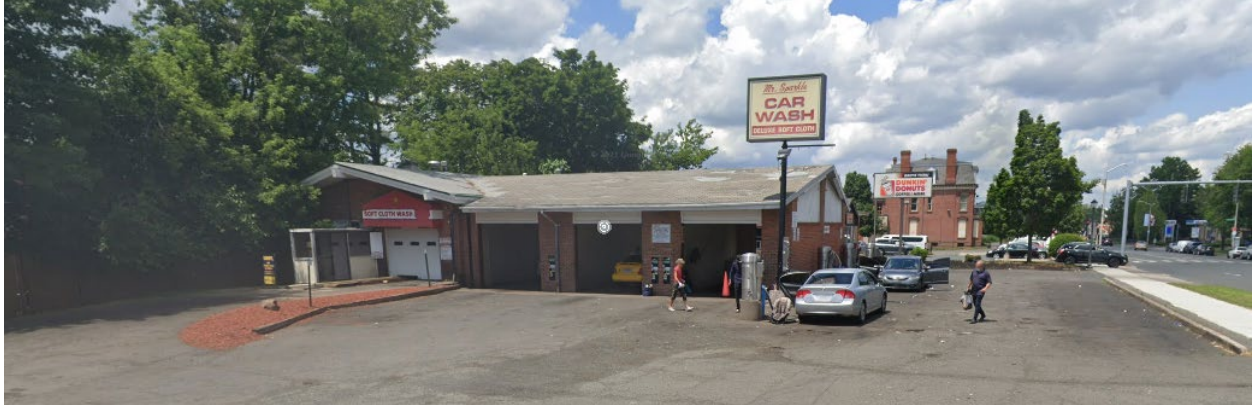
Figure 8. Existing Conditions- 271 Washington St., across Lincoln St. from 289 Washington (Google Maps June 2021)
