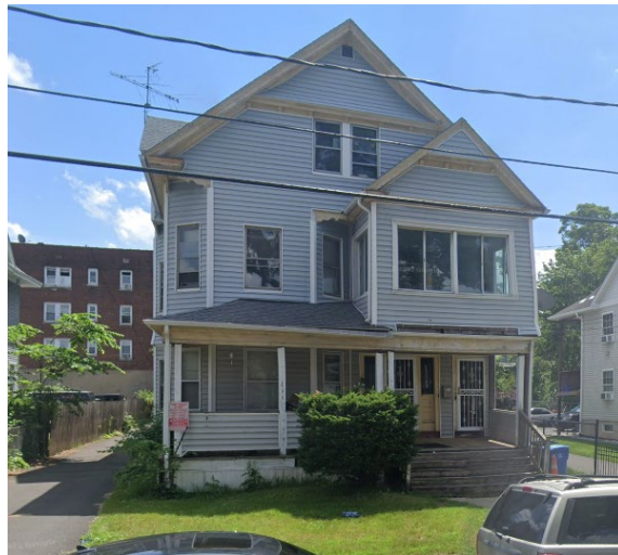
Figure 3. Existing Conditions- 11-13 Lincoln (Google Maps June 2021)
