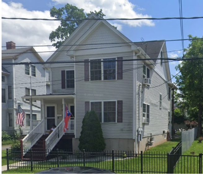
Figure 4. Existing Conditions- 15 Lincoln (Google Maps June 2021)
