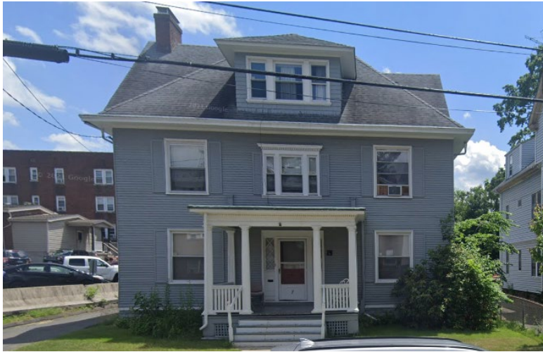
Figure 2. Existing Conditions- 7 Lincoln (Google Maps June 2021)
