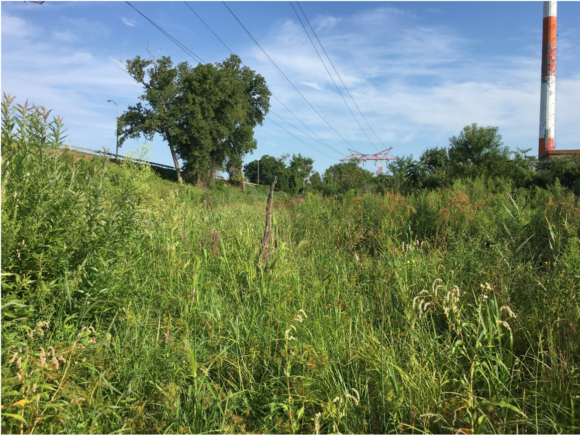
Vegetation growing in the damaged area looking north
