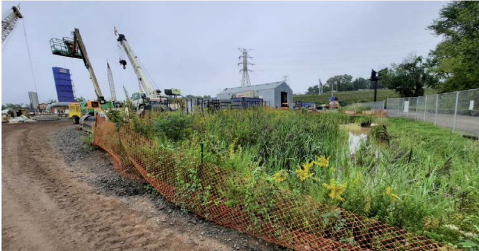
Figure 1. View of main tunnel shaft site at 255 Brainard Rd., taken 9/10/2020.
