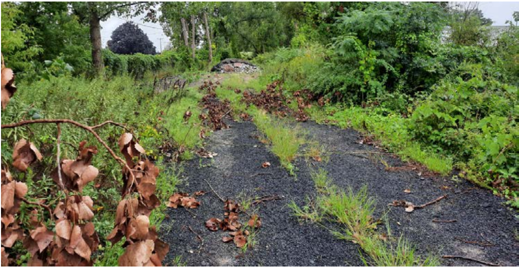
Figure 10. View of apparent clearing and placement of millings within the upland review area on the east side of the watercourse (between Maxim Rd. and the wetlands/watercourse), taken on 9/10/2020.
