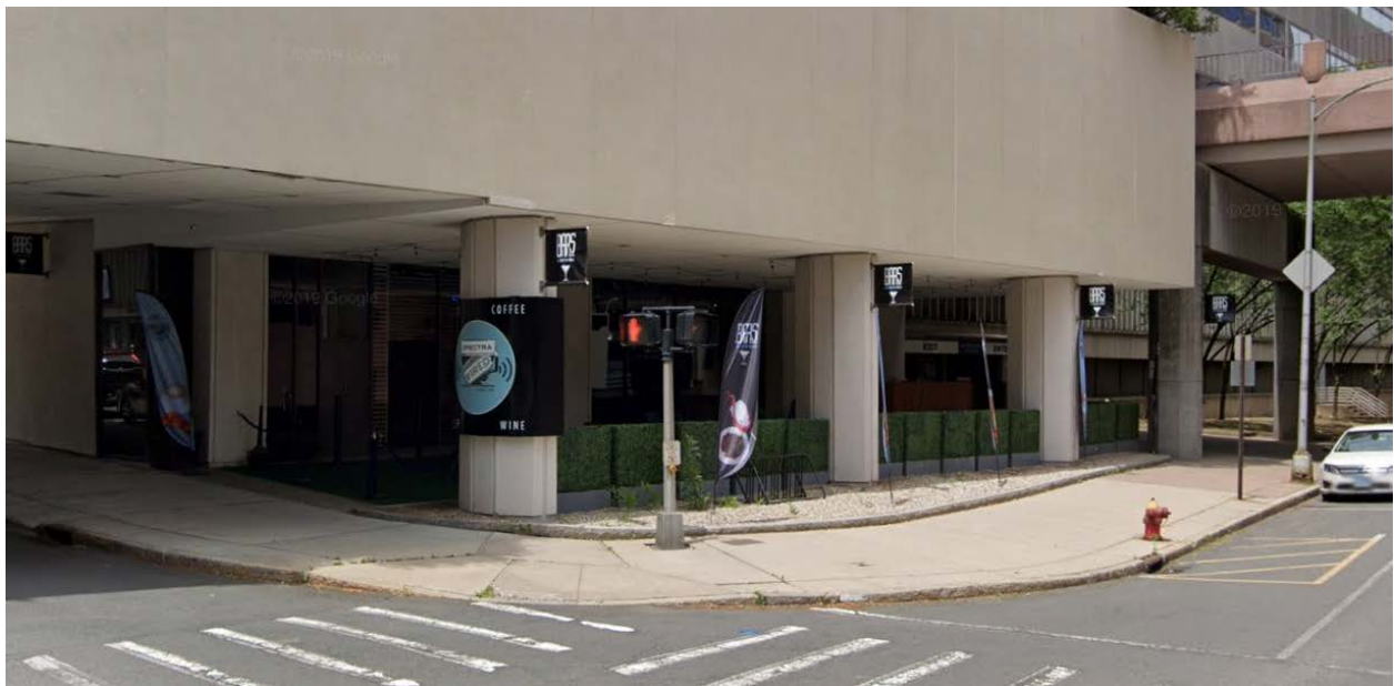
Figure 6. Google Street View, dated June 2019. A closer view of the subject unit from the corner of Columbus and Kinsey depicts the signage of previous tenant and location of the proposed banner signs and refaced cabinet sign. Two of the proposed projecting banner signs will be larger than the current projecting signs and the cabinet sign will be refaced.
